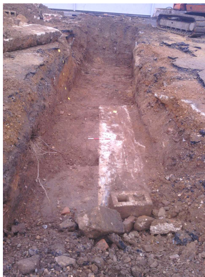
Photograph 1 Trench shot – looking north
