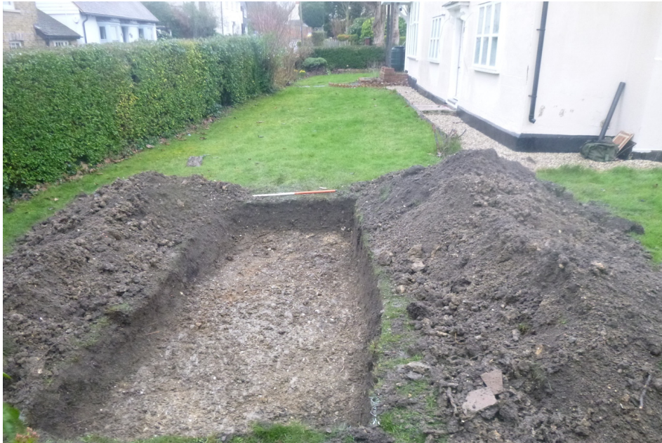
Photograph 1 Trench for underground LPG tank - looking south-west
