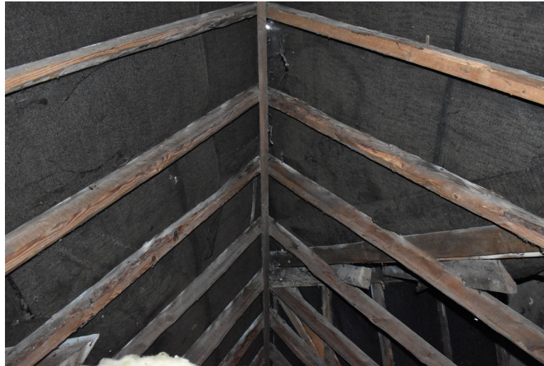
Photograph 11 Roof structure of two-storey range. Photograph taken facing east.
