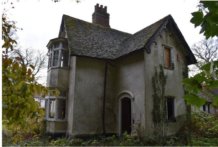
Photograph 8 North elevation of two-storey ranges. Photograph taken facing south-west.
