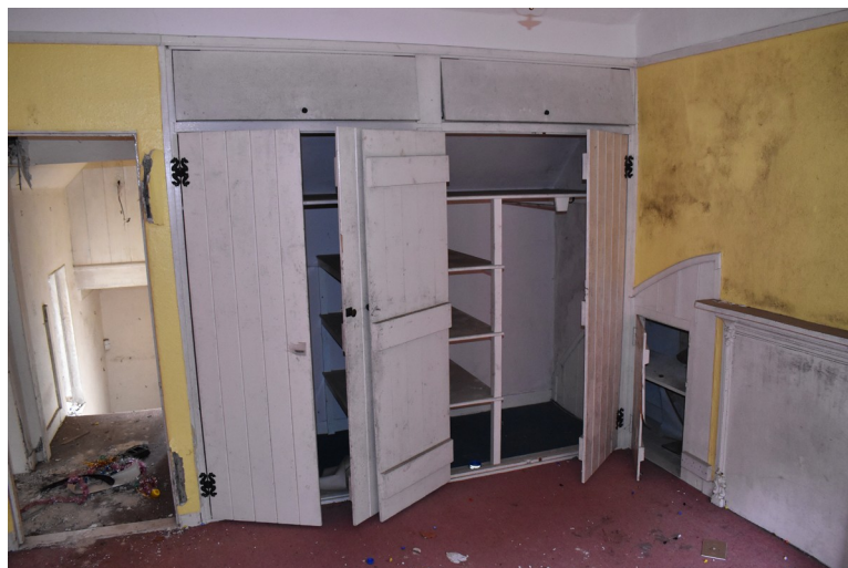
Photograph 25 Interior of room 15, showing inserted cupboards. Photograph taken facing north-west.
