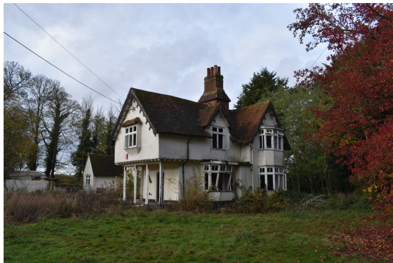
Photograph 2 Modern eastern and southern elevations, showing bay-window extensions, replacement windows and altered chimney. Photograph taken facing north-west.
