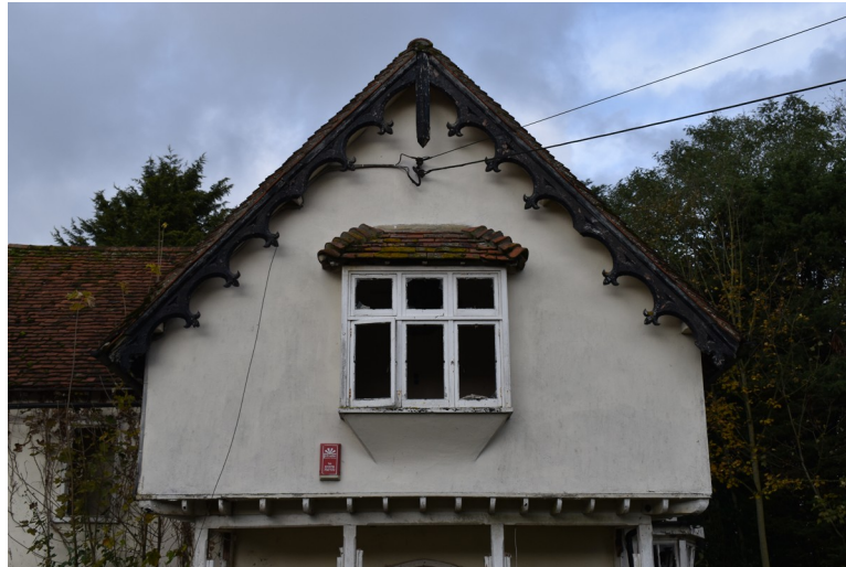
Photograph 6 Detail of south gable-end, showing decorative bargeboards. Photograph taken facing north.
