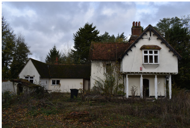
Photograph 4 Southern elevation of building. Photograph taken facing north.
