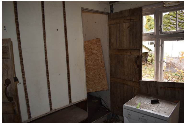
Photograph 20 Interior of room 9, showing doorway accessing staircase. Photograph taken facing south-west.
