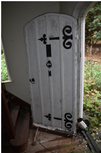
Photograph 9 Exterior door on eastern elevation, with ornate hinges. Photograph taken facing north.
