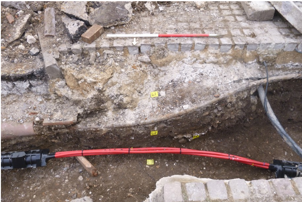
Photograph 3 North-facing section of trench, showing F1. Photograph taken facing south.
