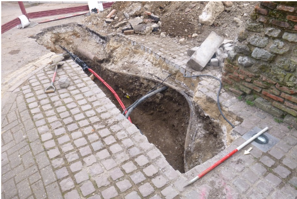
Photograph 1 Trench after excavation and repair of service. Photograph taken facing south-east.
