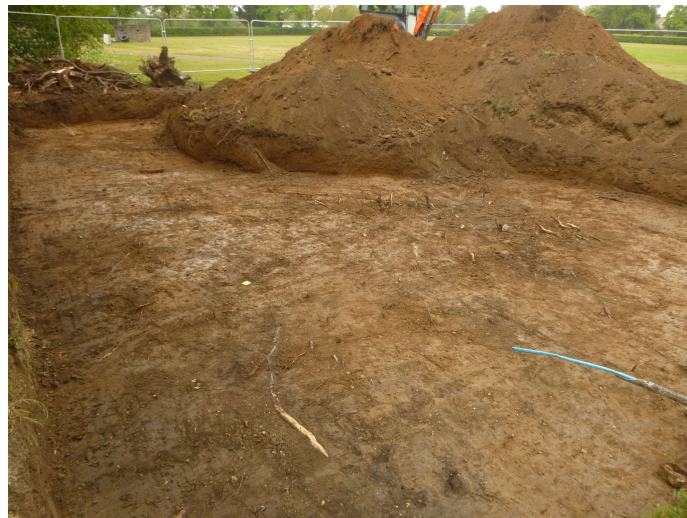
Photograph 1 Excavation area – looking southeast
