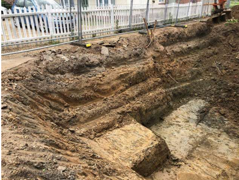
Photograph 3 Site shot following the removal of the petrol tanks
