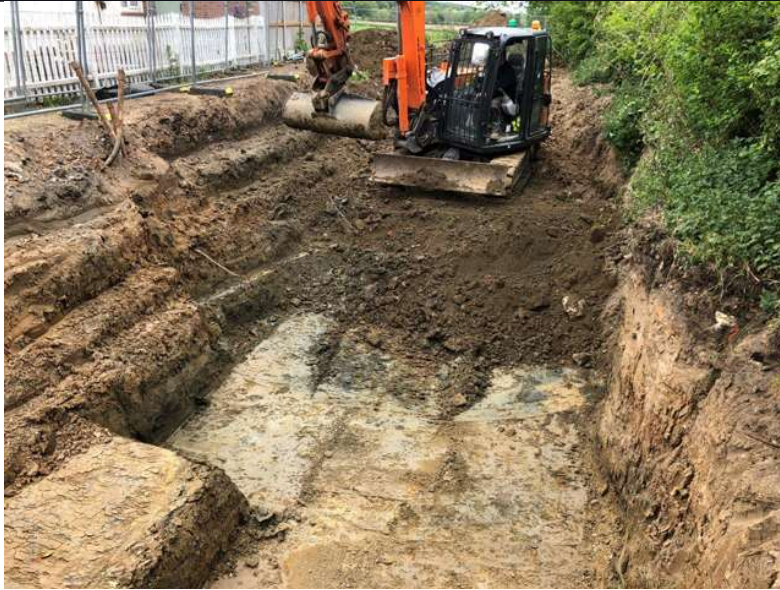
Photograph 2 Site shot following the removal of the petrol tanks
