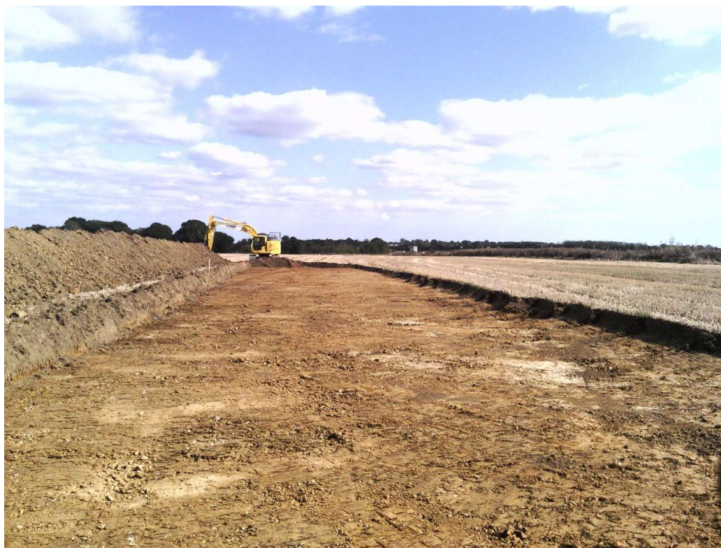
Photograph 1 Phase 3, general site shot, looking E
