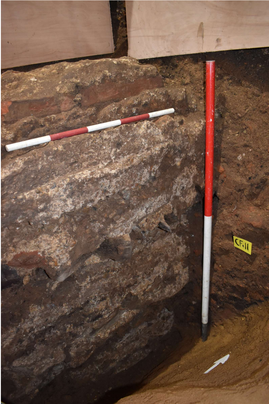
Photograph 11 Pad C, close-up of wall foundation CF8 with construction cut CF11, looking northwest.
