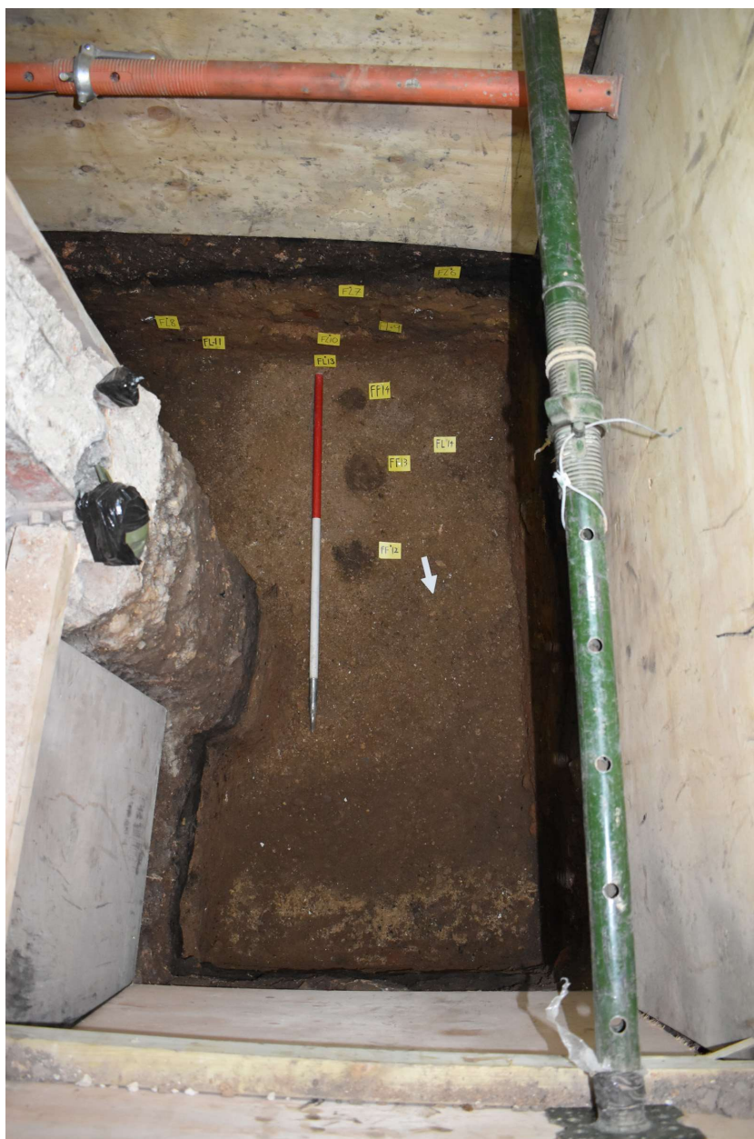
Photograph 13 Pad F, plan of postholes FF12-FF14 cut through metallised surface FL14, looking south.
