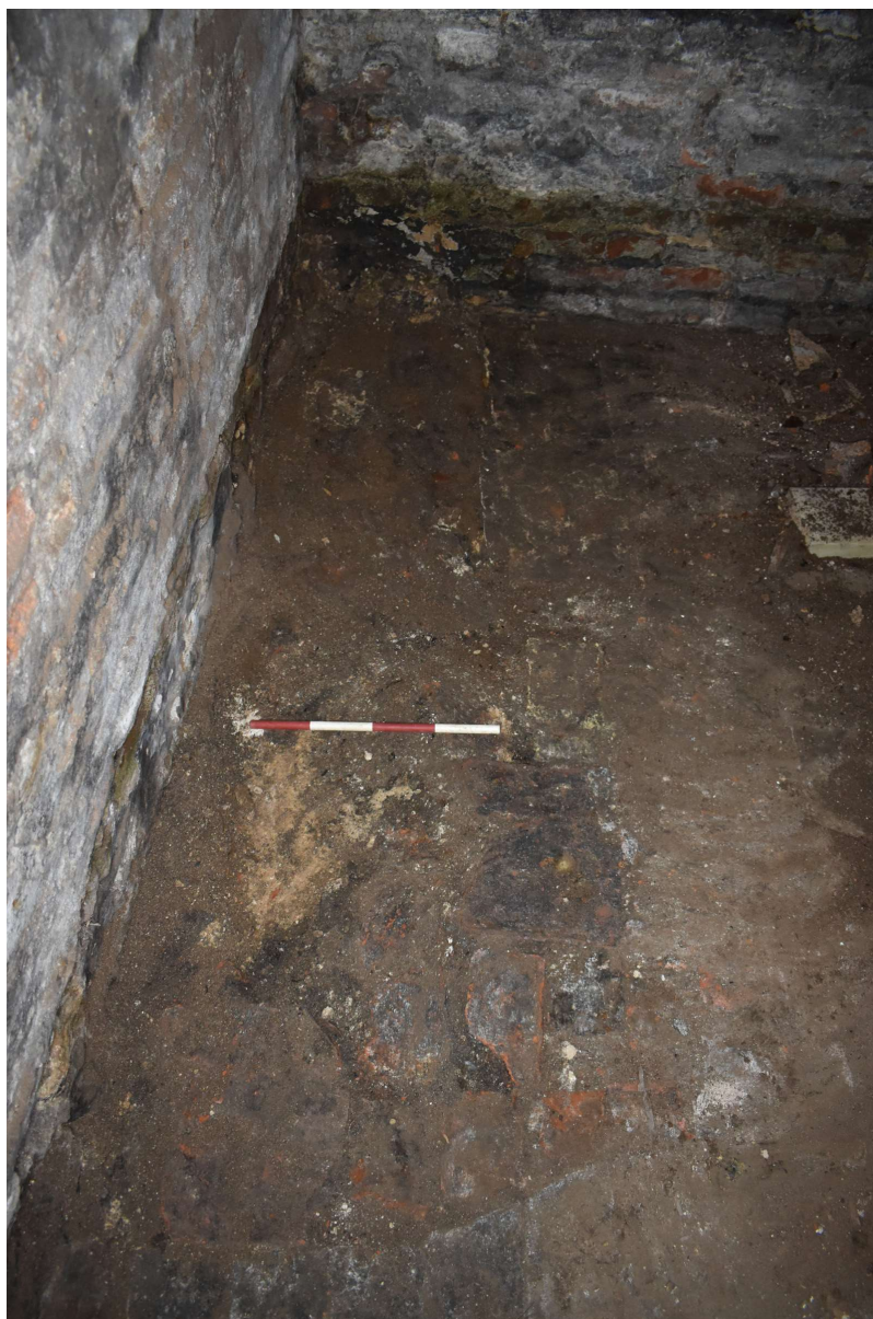
Photograph 30 Roman wall foundation inside the cellar of 6 St Nicholas Street, looking south.
