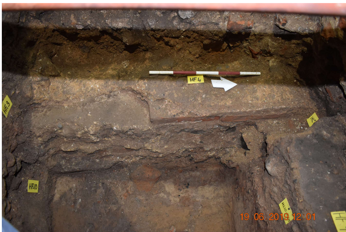
Photograph 26 Pad H, close-up of Roman wall foundation HF4, looking west.
