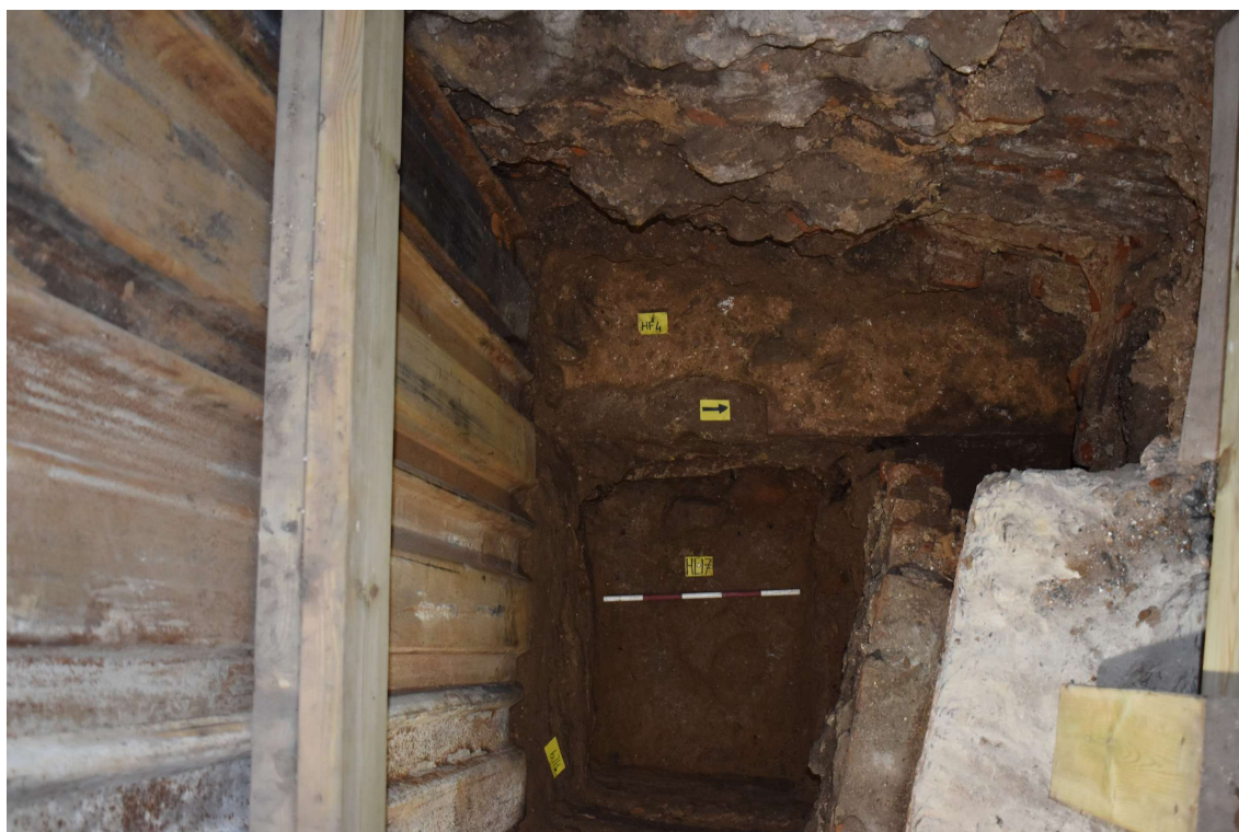
Photograph 24 Pad H, post-medieval cellar wall foundation HF1 built on top of Roman wall foundation HF4, looking west.
