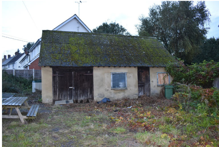
Photograph 2 South-east elevation of the building. Photograph taken facing north-west.
