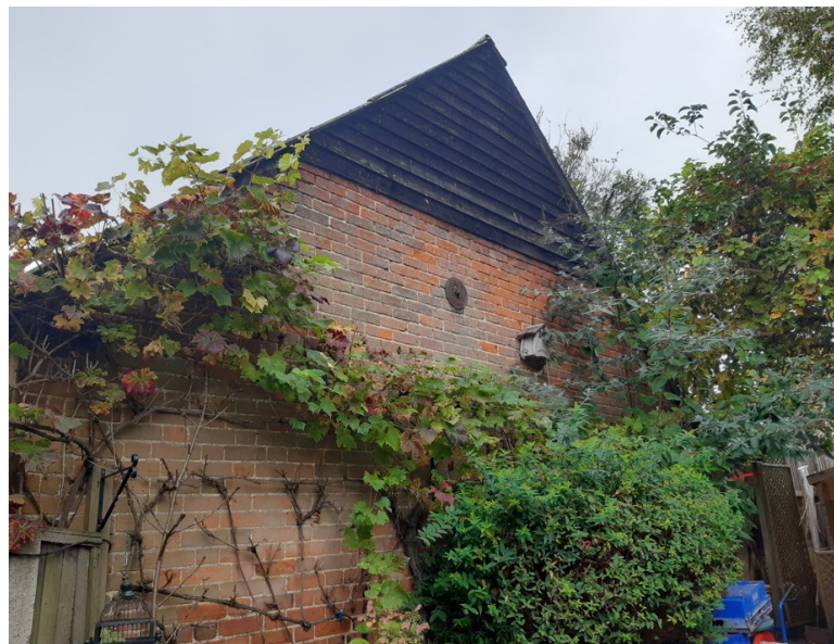
Photograph 3 North-east elevation of building, showing weatherboarding on gable. Photograph taken facing west.
