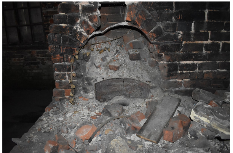
Photograph 8 Detail of opening in chimney of forge, showing firefront. Photograph taken facing north-west.
