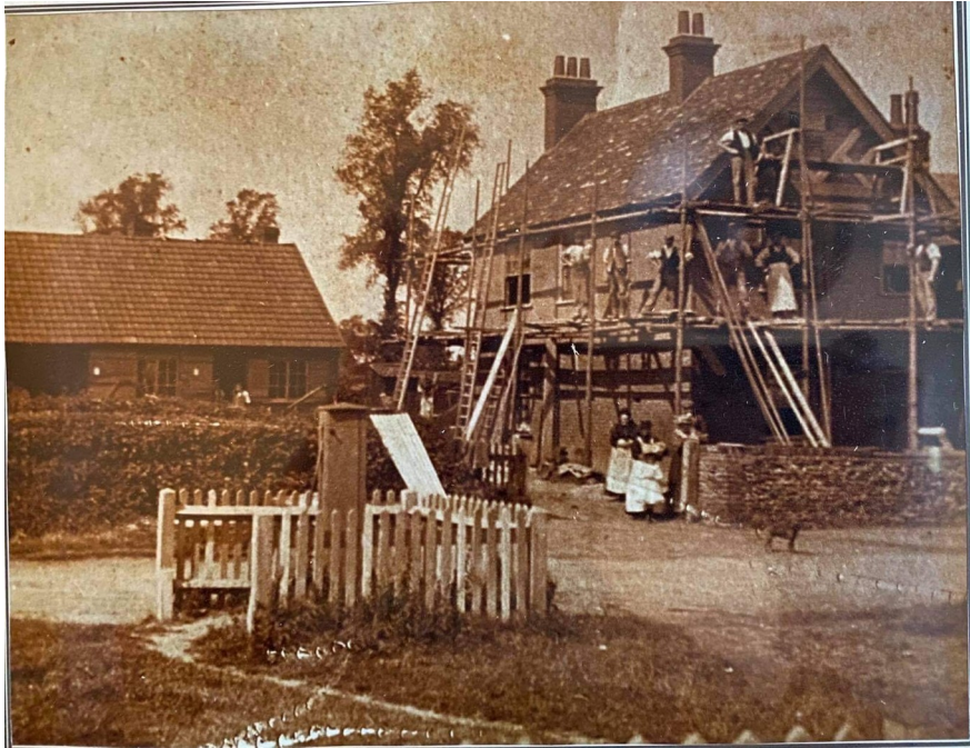
Photograph 1 1903 photograph showing Forge House under construction, with the forge visible to left of frame. Photograph taken facing north-west. Photograph courtesy of residents of Forge House.
