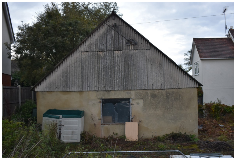
Photograph 5 South-west elevation of building. Photograph taken facing north-east.
