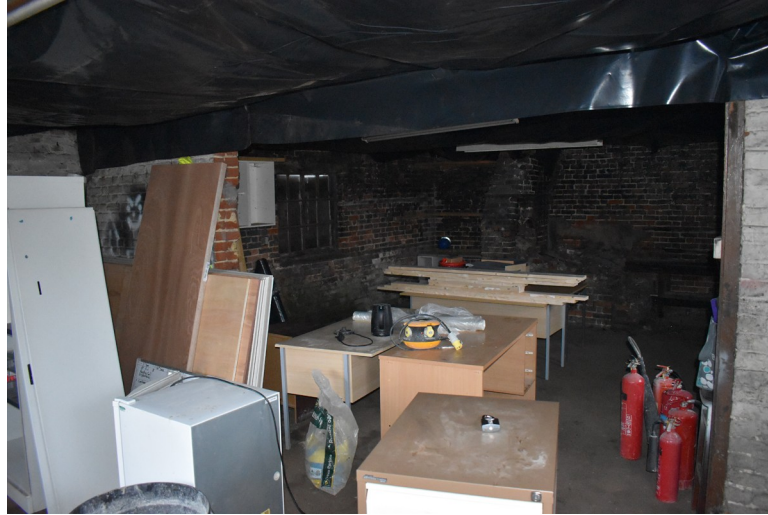
Photograph 12 Interior shot of building. Photograph taken facing north.
