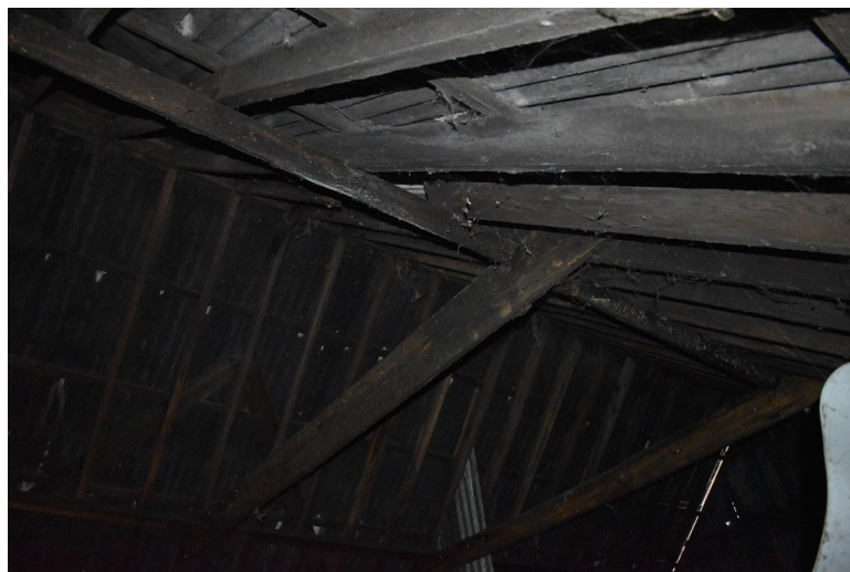
Photograph 11 Detail of roof structure. Photograph taken facing south.
