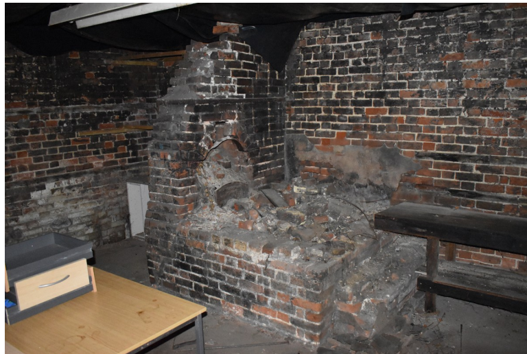
Photograph 6 Detail of forge within the building. Soot blackening visible on walls. Photograph taken facing north.
