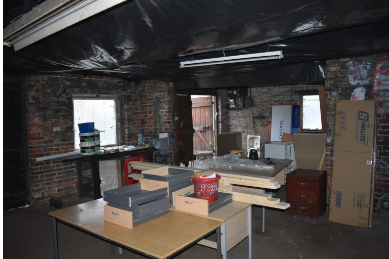
Photograph 9 Interior of building showing modern additions and furniture. Photograph taken facing south.
