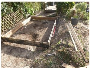
Photograph 1 Raised foundation of summerhouse visible prior to pouring of concrete. Photograph taken facing north-west. Flowerbed to be lowered visible on right. Photograph taken facing south-east.
