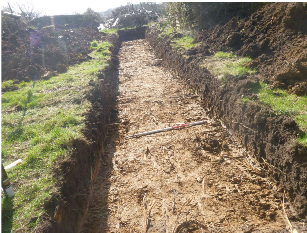
Photograph 2 Trench 2, looking southwest
