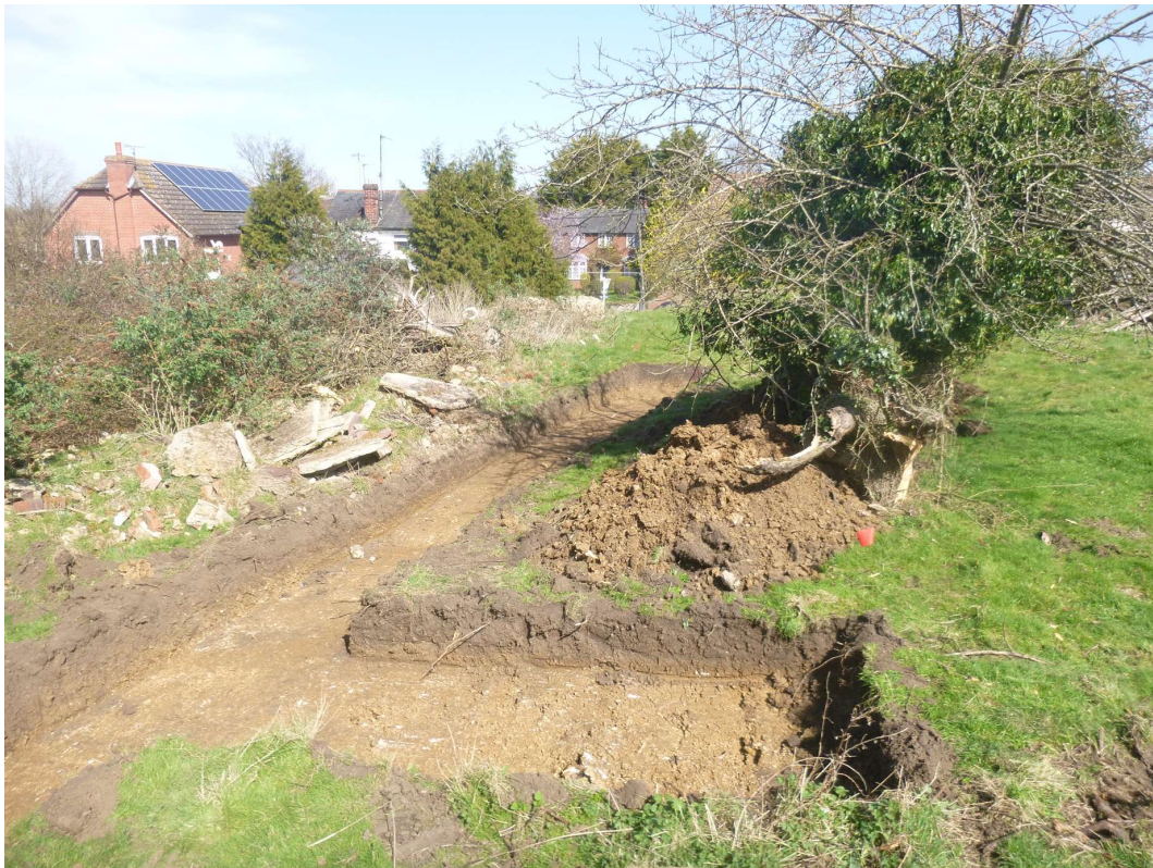
Photograph 1 Trench 1, looking northeast
