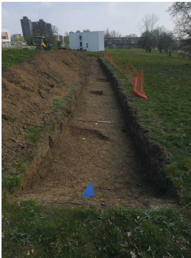
Photograph 4 T3 trench shot – looking southeast
