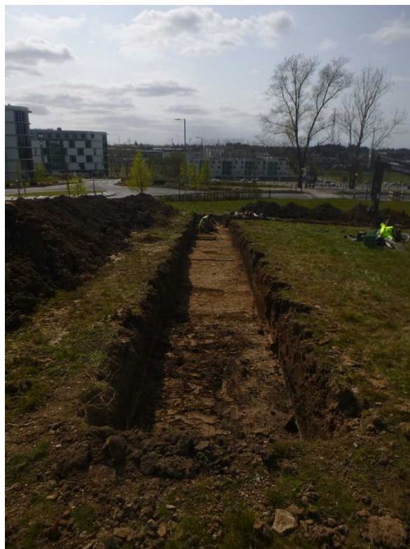
Photograph 7 T6 trench shot – looking southwest
