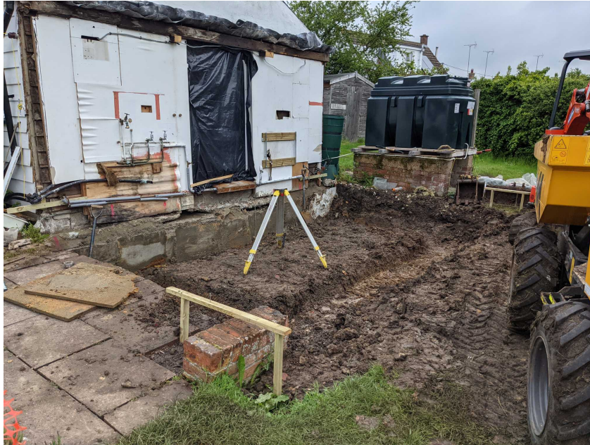
Photograph 1 Extension foundation trenches - view NE
