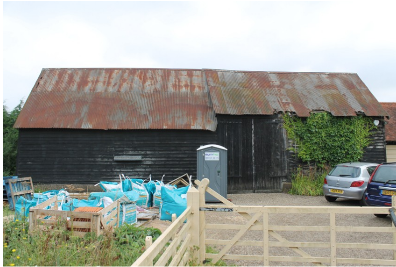
Photograph 2 South-west elevation of the barn. Photograph taken facing north-east.
