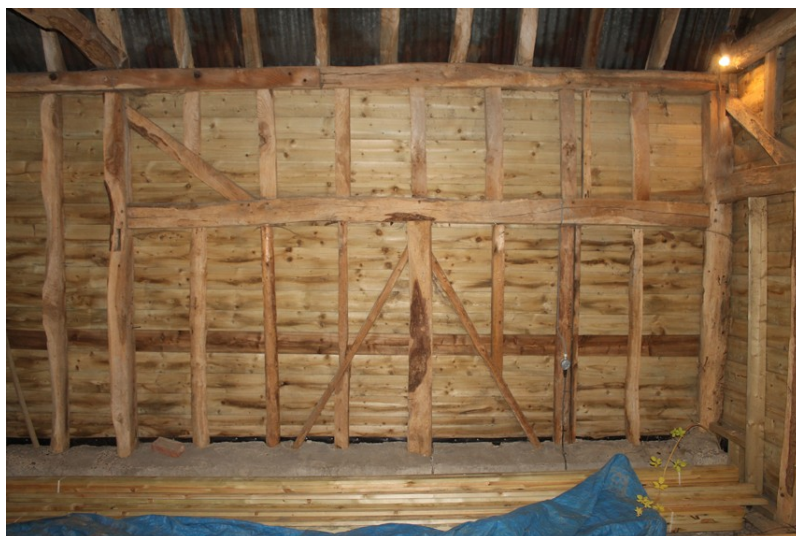
Photograph 5 Detail of southern elevation of bay 1, showing girding-beam and nailed together lower-register. Photograph taken facing south-west.
