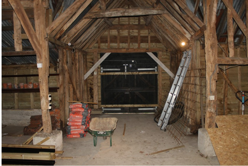
Photograph 19 Detail of midstrey, showing barn doors. Photograph taken from bay 4, facing north-east.
