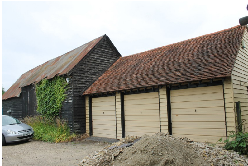
Photograph 3 South-east elevation of the barn, with modern garage. Photograph taken facing north-east.
