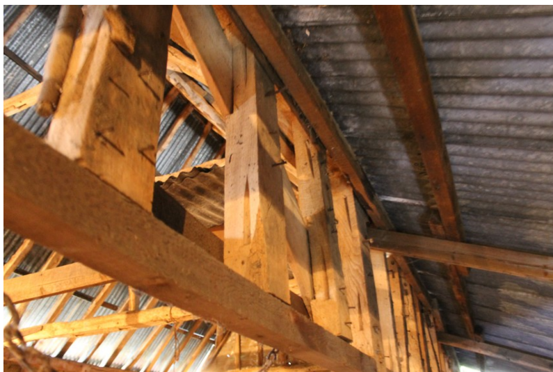
Photograph 10 Detail of studs in bay 2, showing grooves. Photograph taken from western lean-to, facing west.
