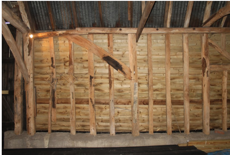
Photograph 13 Southern elevation of bay 3, showing arched brace. Photograph taken facing south-west.
