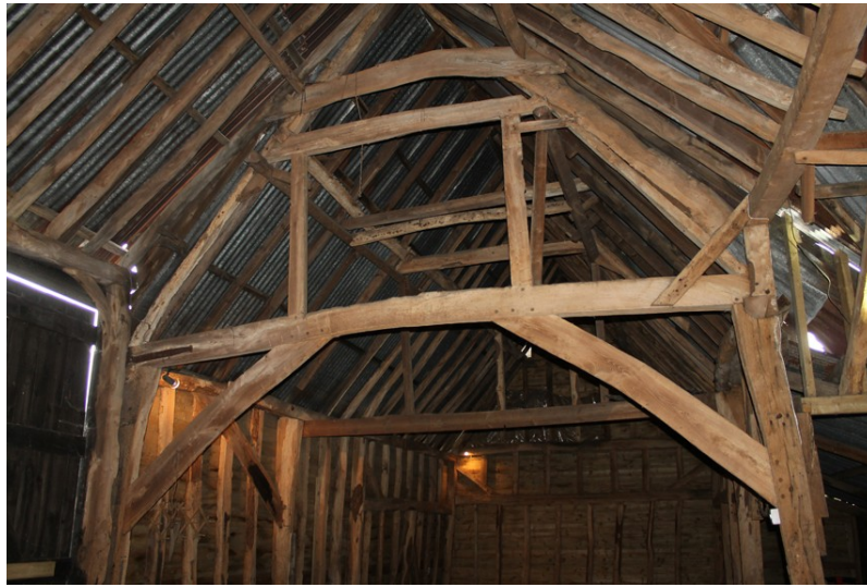
Photograph 4 Detail of truss between bays 3 and 4. Photograph taken facing west.
