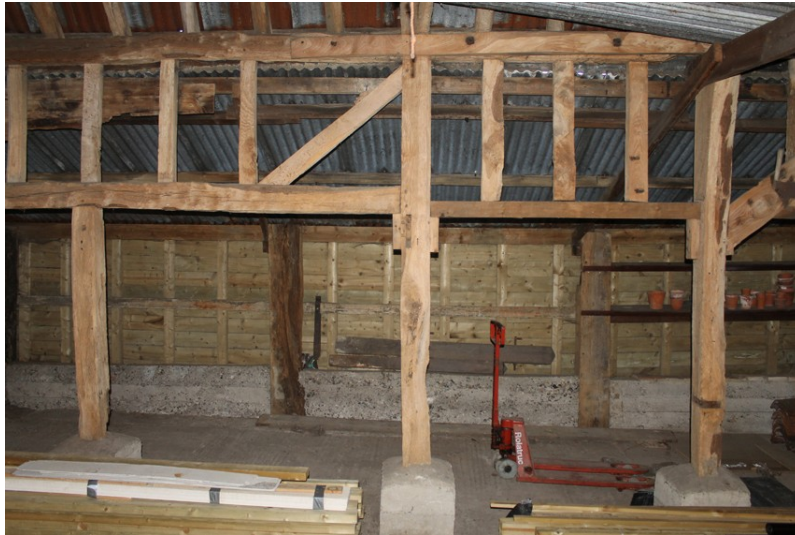
Photograph 9 Detail of northern principal-post between bays 1 and 2, showing frames on either side. Photograph taken facing north-east.
