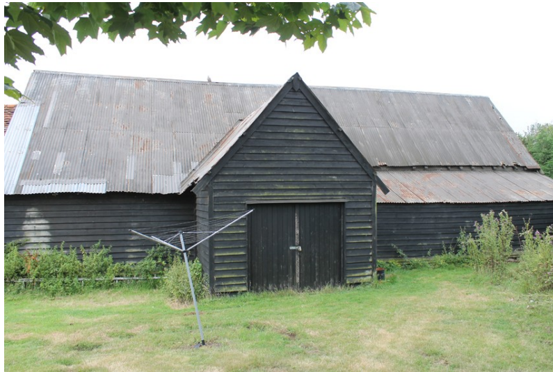
Photograph 1 North-east elevation of barn, showing midstrey and lean-tos. Photograph taken facing south-west.
