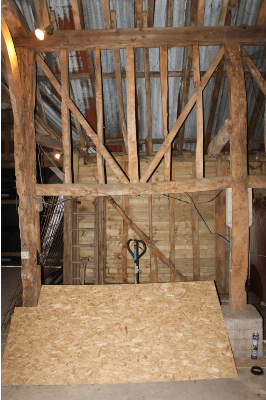
Photograph 16 Northern elevation of bay 5. Photograph taken facing north-east.
