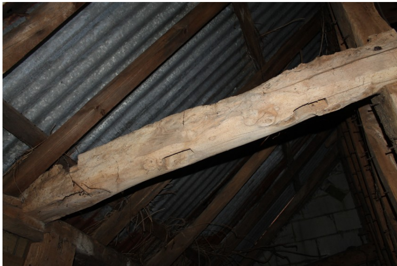
Photograph 20 Detail of re-used beam in eastern lean-to, showing empty mortices. Photograph taken facing east.
