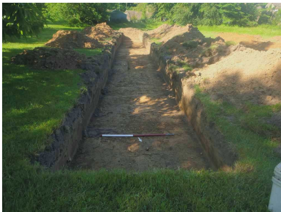
Photograph 4 T15 trench shot – looking south-south-west
