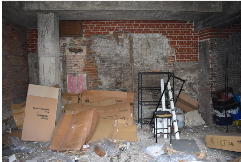
Photograph 7 Detail of section 6 behind 35-36 St John's Street, showing multiple phases of brickwork. Visible in bottom right of frame is exposed septaria and mortar core. Photograph taken facing north.
