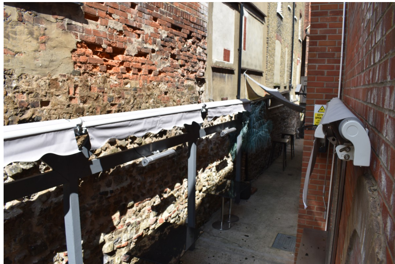
Photograph 12 Section 8 of wall, projecting to the east. Photograph taken facing north-east.
