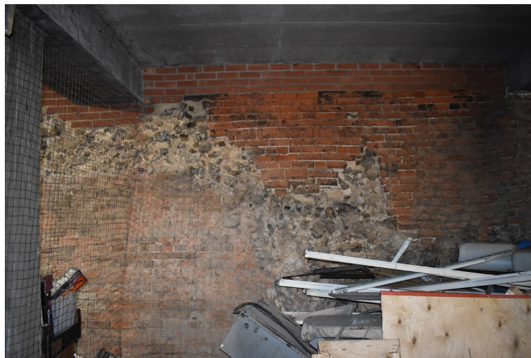
Photograph 6 Detail of section 6, showing modern brickwork alongside re-used septaria. Photograph taken facing north.
