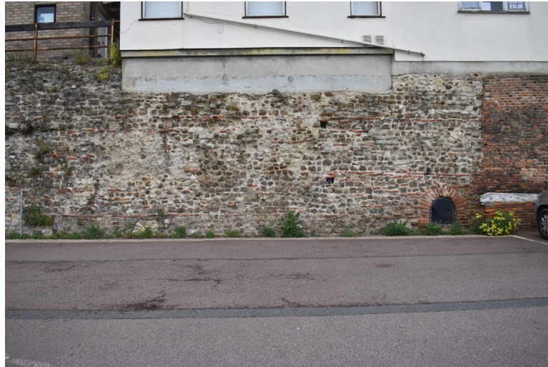
Photograph 11 Detail of section 7, showing medieval 'putlog' holes and refaced Roman culvert. Photograph taken facing north.
