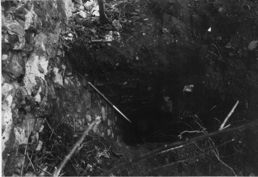
Photograph 4 Detail of test-pit from 1991 showing battered medieval face of town wall. Photograph taken facing east.
