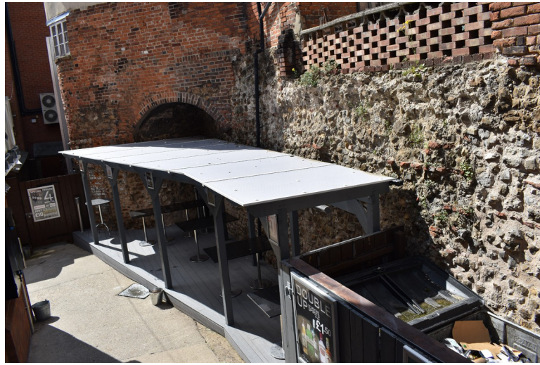
Photograph 13 Section 8 of wall, with Bastion 6 visible at rear. Photograph taken facing north-west.
