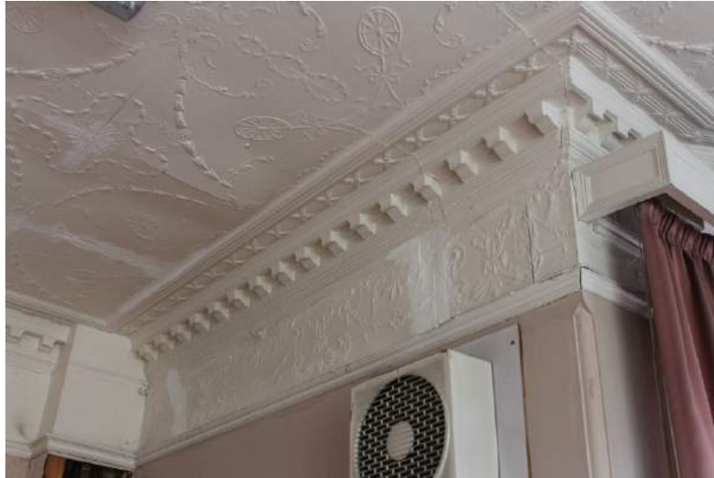
Photograph 21 Detail of cornicing and ceiling paper in room 6. Photograph taken facing east.
