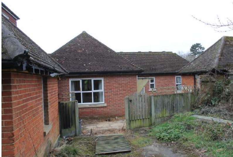
Photograph 16 Modern extension on north-east elevation. Photograph taken facing south-west.
