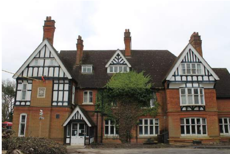
Photograph 11 North-east elevation of Foley House. Photograph taken facing south-west.
