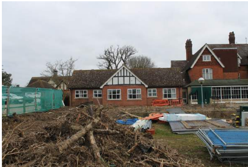
Photograph 7 Modern extension at western end of south-west elevation. Photograph taken facing north-east.
