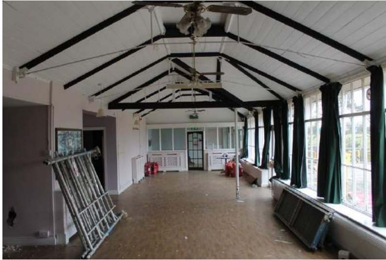
Photograph 30 Interior of conservatory. Photograph taken facing south-east.
