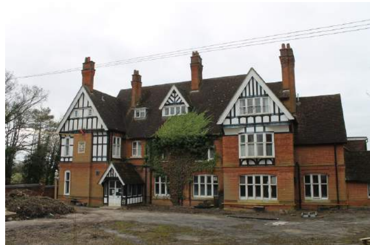
Photograph 2 Present day north-east elevation of Foley House. Photograph taken facing south-east.
