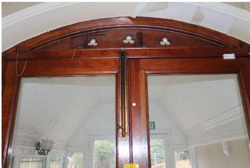
Photograph 25 Detail of ventilation panel on door between rooms 12 and 13. Photograph taken facing north-east.
