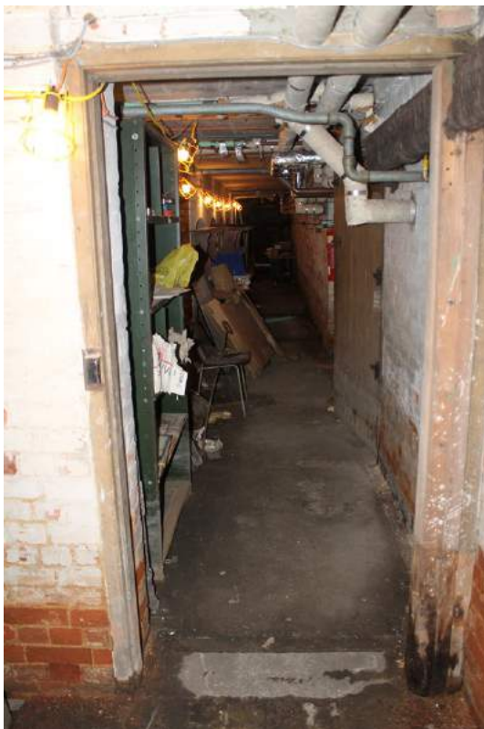
Photograph 18 Basement corridor. Photograph taken facing north-west.
