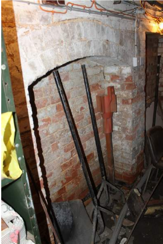
Photograph 19 Detail of brick arch in basement. Photograph taken facing west.
