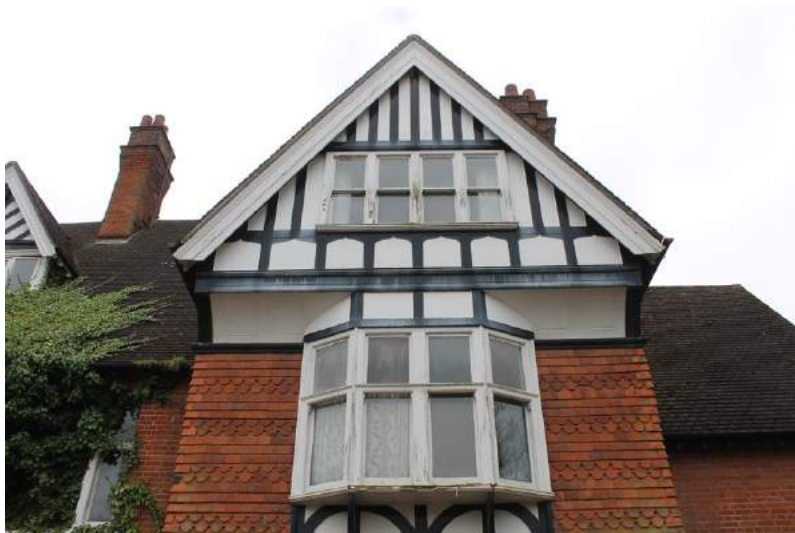
Photograph 14 Detail of projecting bay at west end of north-east elevation, showing oriel window and jettied gable. Photograph taken facing south-west.
