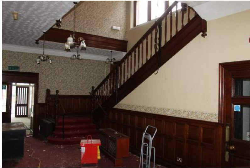
Photograph 23 Room 8, showing original staircase. Photograph taken facing west.
