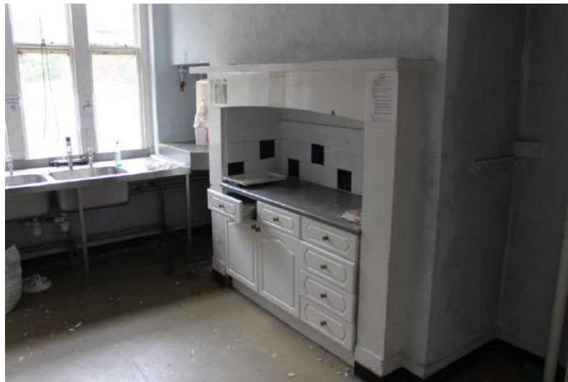
Photograph 29 Alcove in room 18 that would have housed original range in kitchen. Photograph taken facing east.
