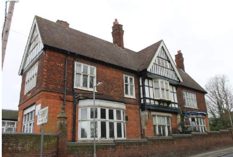
Photograph 9 South-east elevation of Foley House. Photograph taken facing north.
