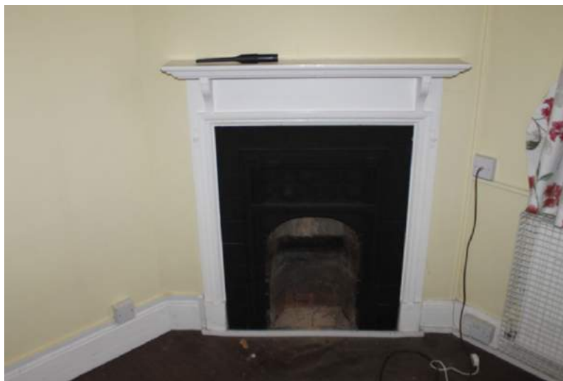
Photograph 33 Original fireplace in room 85. Photograph taken facing south.
