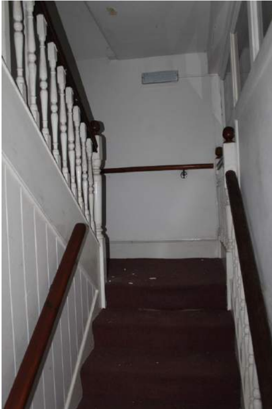
Photograph 32 Detail of staircase in room 23. Photograph taken facing north-west.
