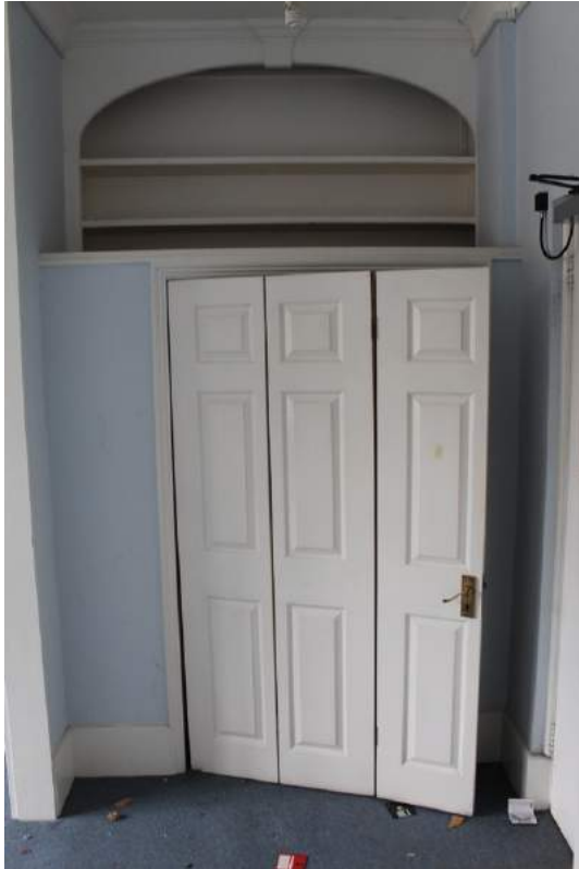
Photograph 28 Detail of original display cupboard in room 16, and later modern cupboard partially obscuring it. Photograph taken facing south-east.
