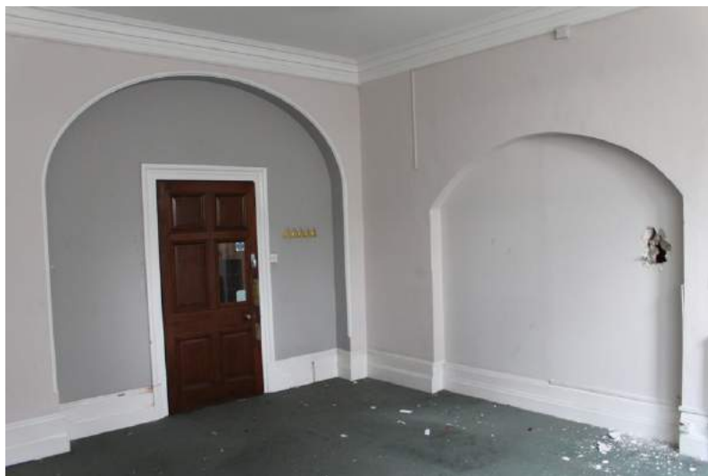
Photograph 20 Detail of blocked arches leading out of room 7 into rooms 8 (left) and 11 (right). Photograph taken facing north.
