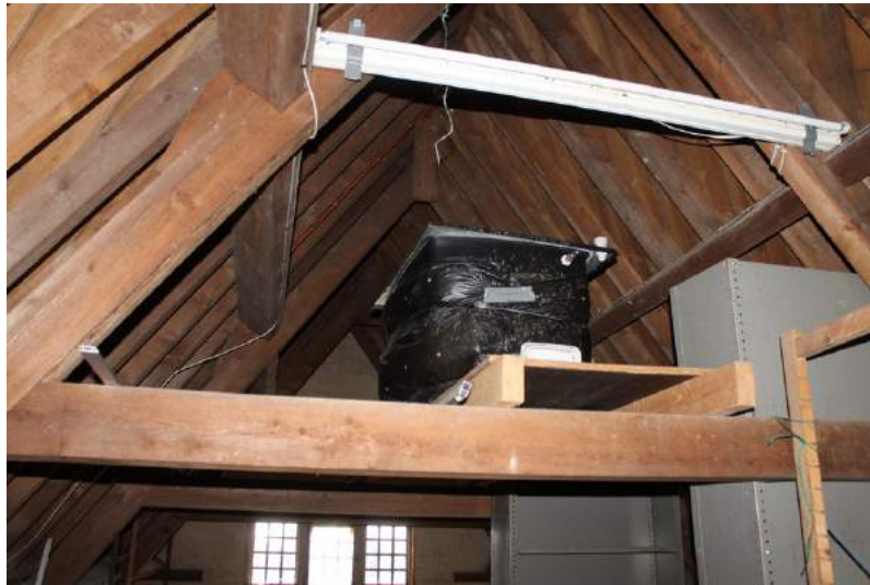
Photograph 37 Room 90, showing exposed roof timbers. Photograph taken facing south-west.
