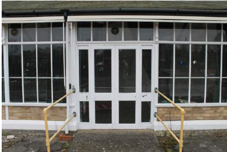
Photograph 6 Original opening into conservatory (with modern doors). Modern brickwork visible below. Photograph taken facing north-east.
