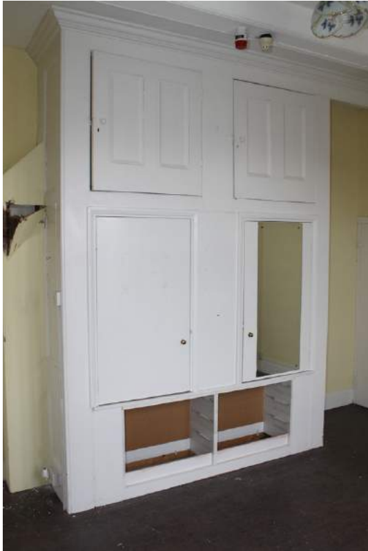
Photograph 34 Detail of cupboard in room 85. Photograph taken facing east.
