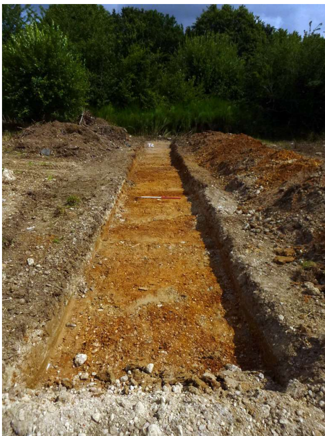
Photograph 1 Trench T2, looking northeast
