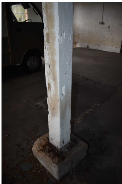
Photograph 14 Empty mortices on post in Room 1 – view south-west.
