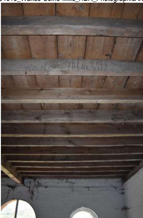
ECC4613_Photo... Baltic timber mark on joist supporting Room 6 - view south.
