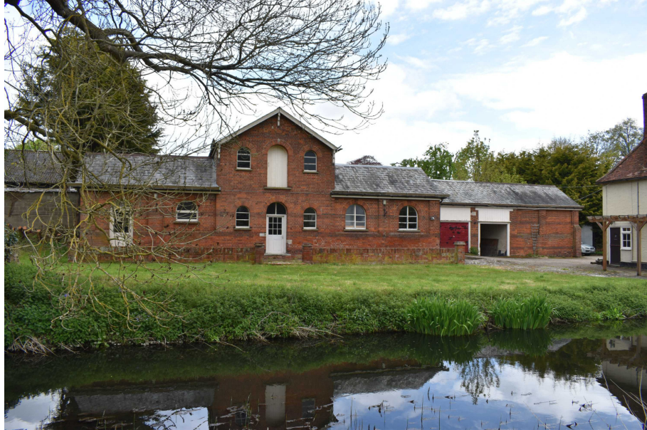
Photograph 1 South elevation of coach house - view north.
