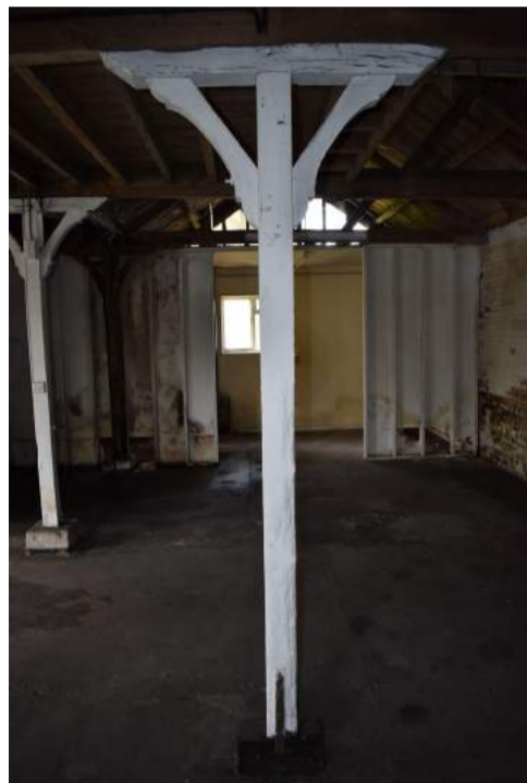
ECC4613_Photograph_052 Original (but relocated) post in Room 1 - view west.
