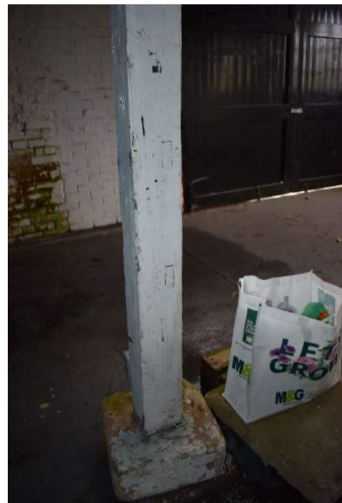
ECC4613_Photograph_066 Sawn off tenons in the mortices on post in Room 1, would have originally supported division.
