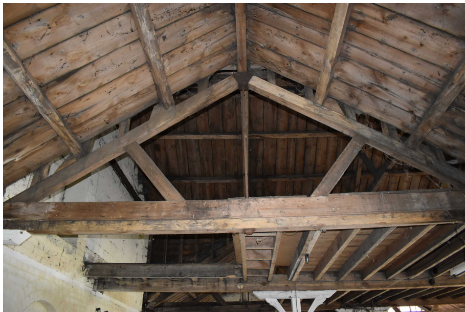
Photograph 16 Truss above western end of Room 1 - view east.
