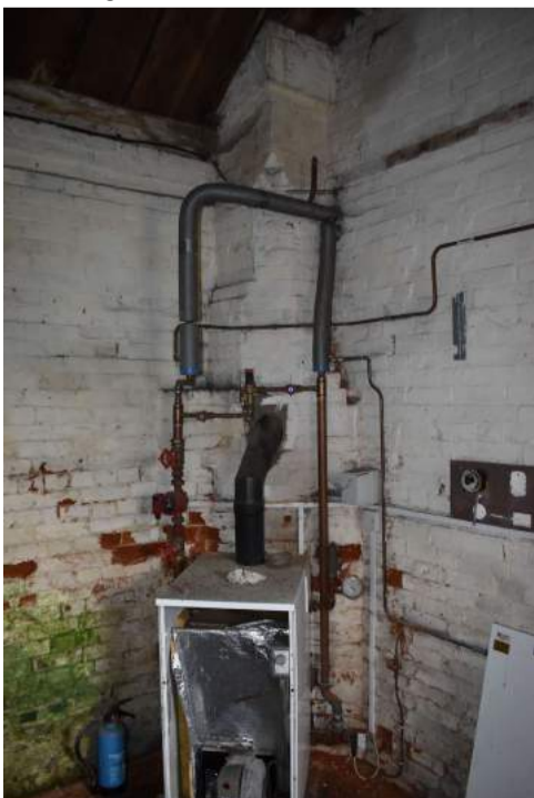
ECC4613_Photograph_082 Detail of original fireplace and chimney-stack in Room 2, with modern addit...
