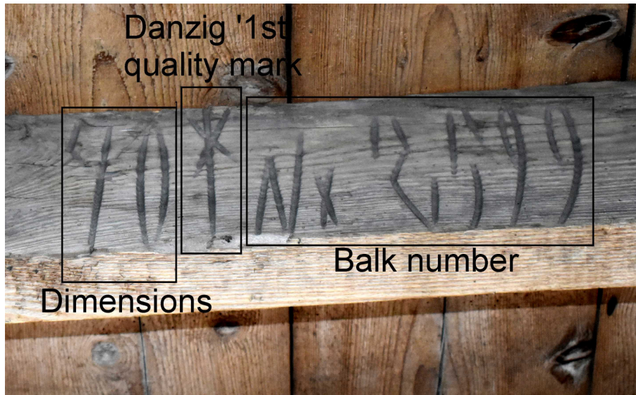
Photograph 22 Example of a Baltic timber mark. Photograph enhanced for legibility.
