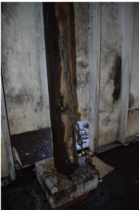
ECC4613_Photograph_068 Detail of mortices in original post in Room 1 - view north-west.
