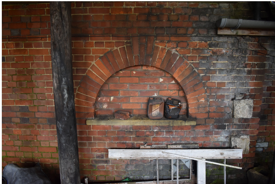
Photograph 10 Blocked window on the north elevation of the cross-wing to the main range – view south.
