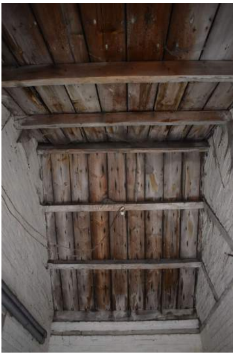
ECC4613_Photograph_013 Roof above Room 4 - view north.
