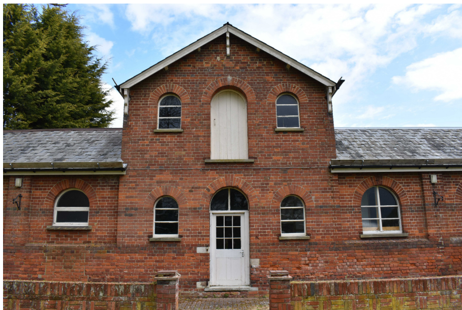
Photograph 2 South elevation of the main range - view north.
