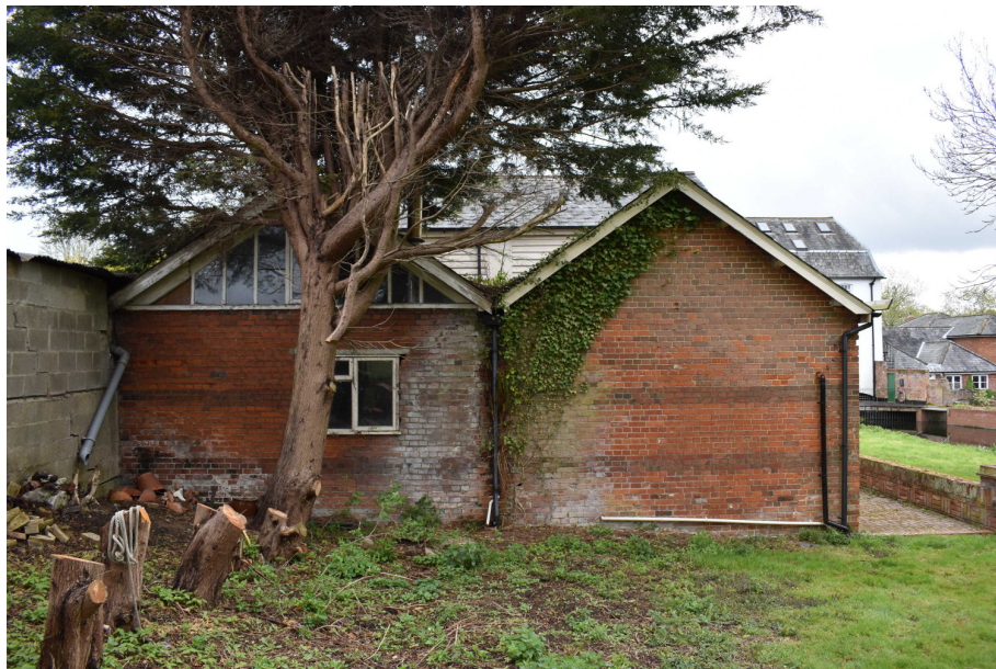
Photograph 12 West elevation of the main range - view east.
