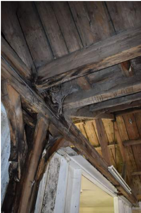
ECC4613_Photograph_125 Location of Baltic timber mark on joist supporting Room 6 - view north-west.
