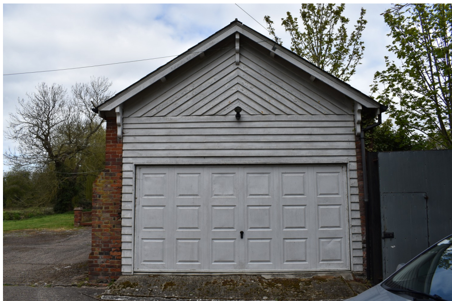
Photograph 9 East elevation of the secondary range – view west.
