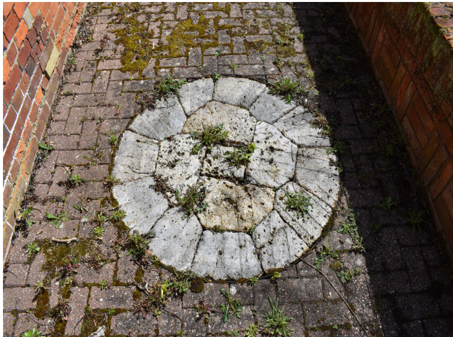
Photograph 7 Detail of millstone fragments in brick floor in front of the main range to the coach house - view east.
