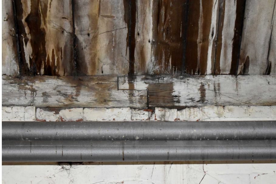
Photograph 21 Detail of northern wall-plate scarf joint in Room 3 - view north.
