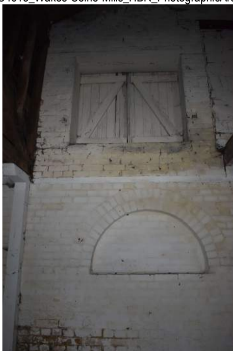
ECC4613_Photograph_050 Room 1, showing blocked window and inserted pitching-door on north elev...
