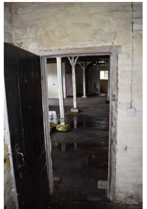
ECC4613_Photograph_084 Doorway into Room 1 from Room 2, with arch above - view east.
