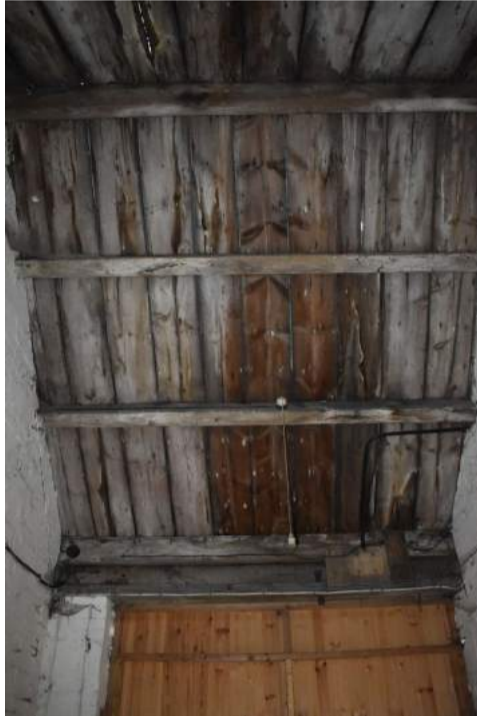
ECC4613_Photograph_089 Southern roof pitch above Room 3 - view south.
