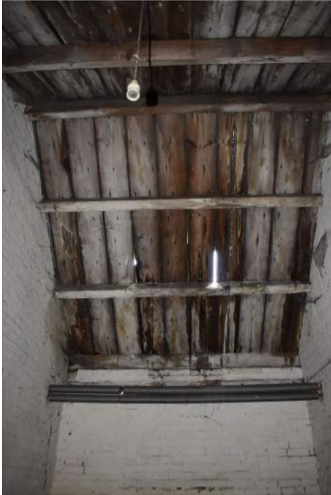
ECC4613_Photograph_088 Northern roof pitch above Room 3 - view north.
