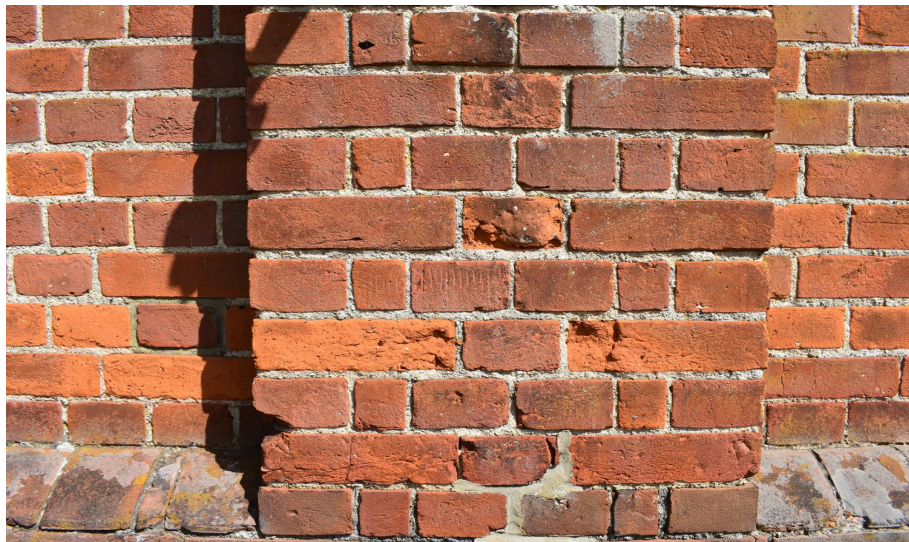
Photograph 5 Detail of graffiti on south elevation of the main range – view north
