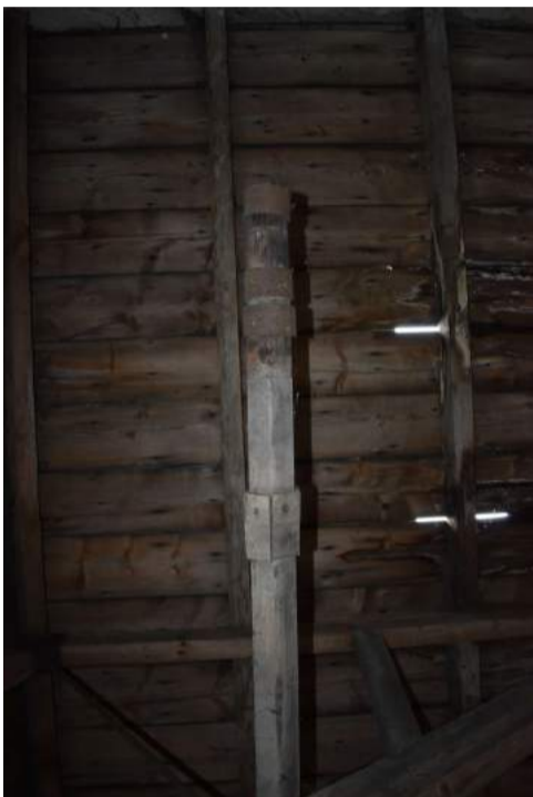
ECC4613_Photo... Detail of large timber that was originally from mill machinery supported on ti...
