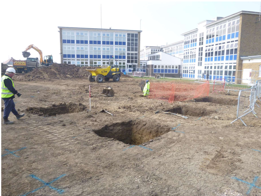
Photograph 2 Working shot of foundation pad excavations, looking southwest
