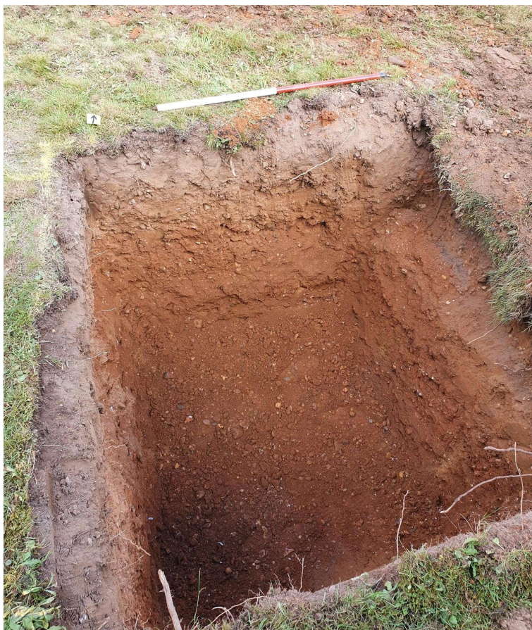
Photograph 3 Excavated soakaway, looking north
