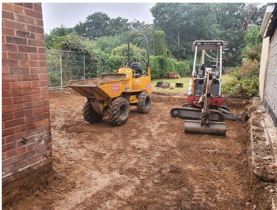
Photograph 1 Area of site reduced prior to excavation, looking roughly west
