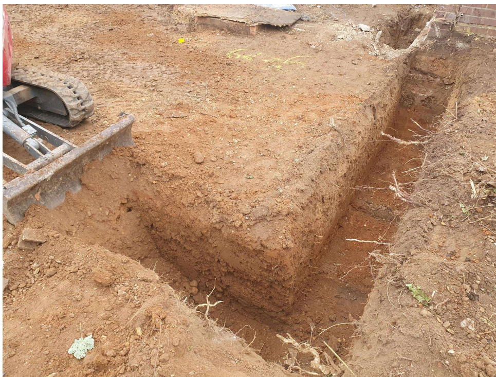
Photograph 2 Excavation of main footings, looking roughly east
