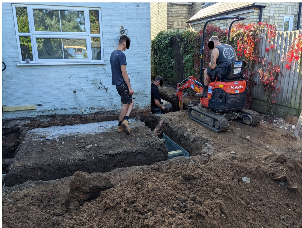
Photograph 2 Rear and partial side foundation trenches, looking south
