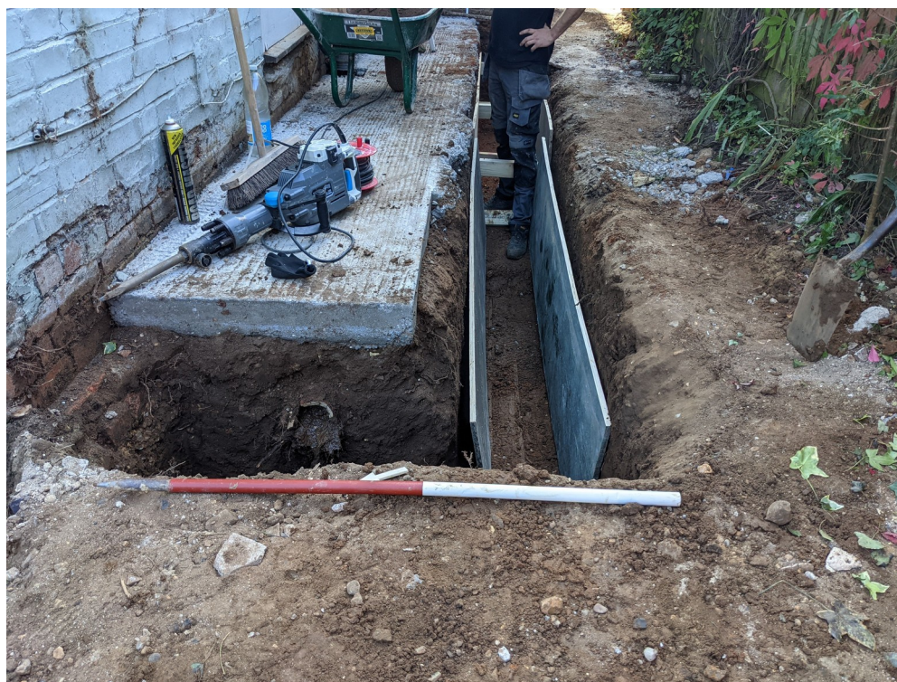
Photograph 3 Side foundation trench, looking south-east
