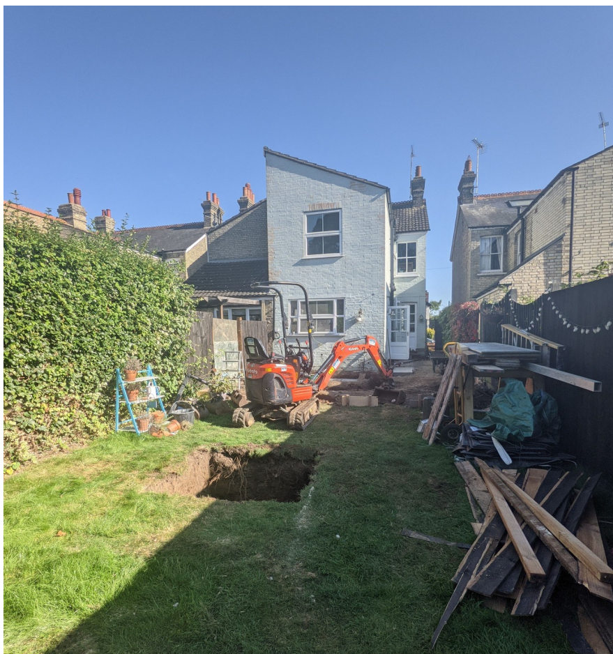
Photograph 4 Soakaway to rear of house, looking south-east
