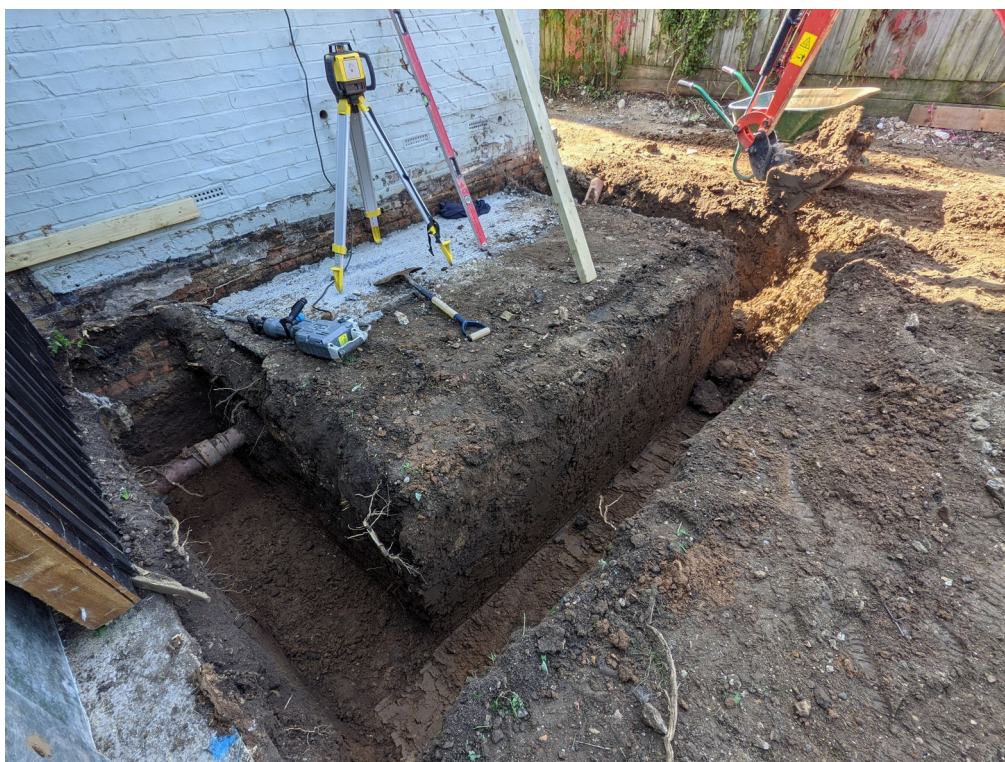
Photograph 1 Rear foundation trenching, looking south
