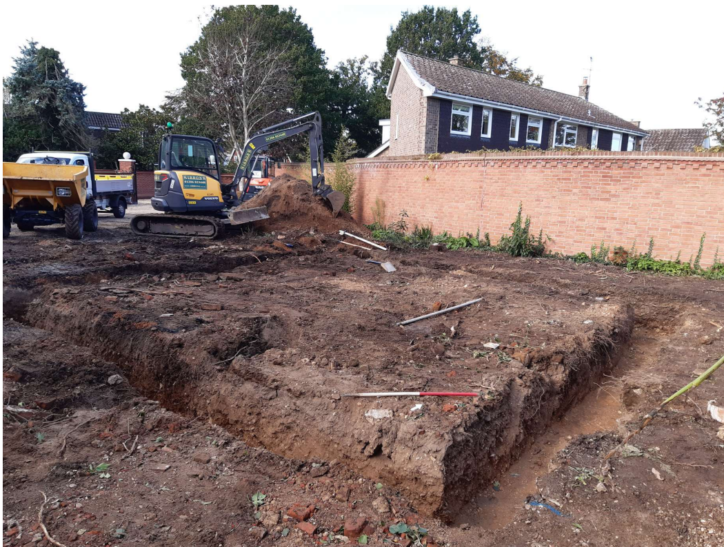
Photograph 1 Foundation trench, looking northwest
