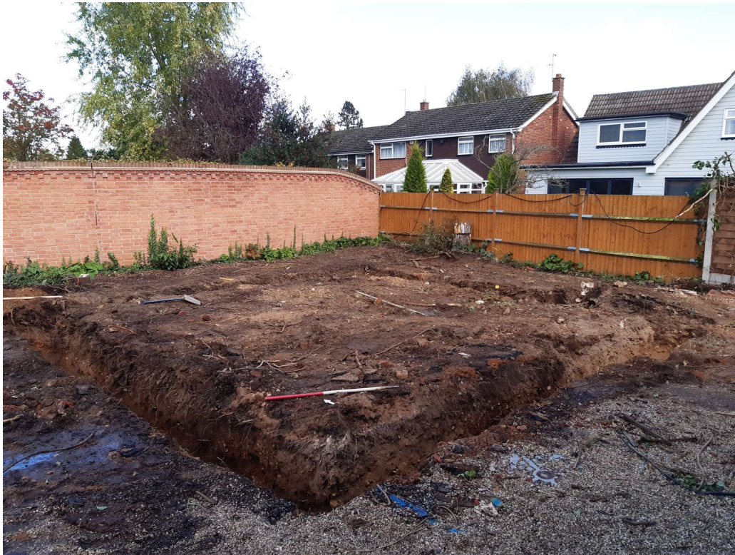
Photograph 2 Foundation trench, looking northeast
