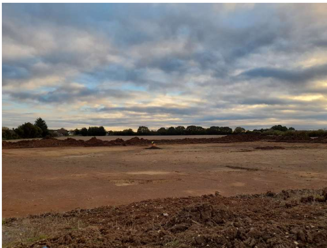
Photograph 1 Site shot, looking south-east
