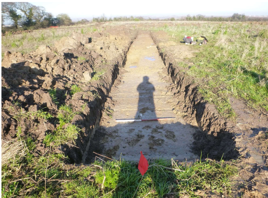
Photograph 8 T48 trench shot – looking north
