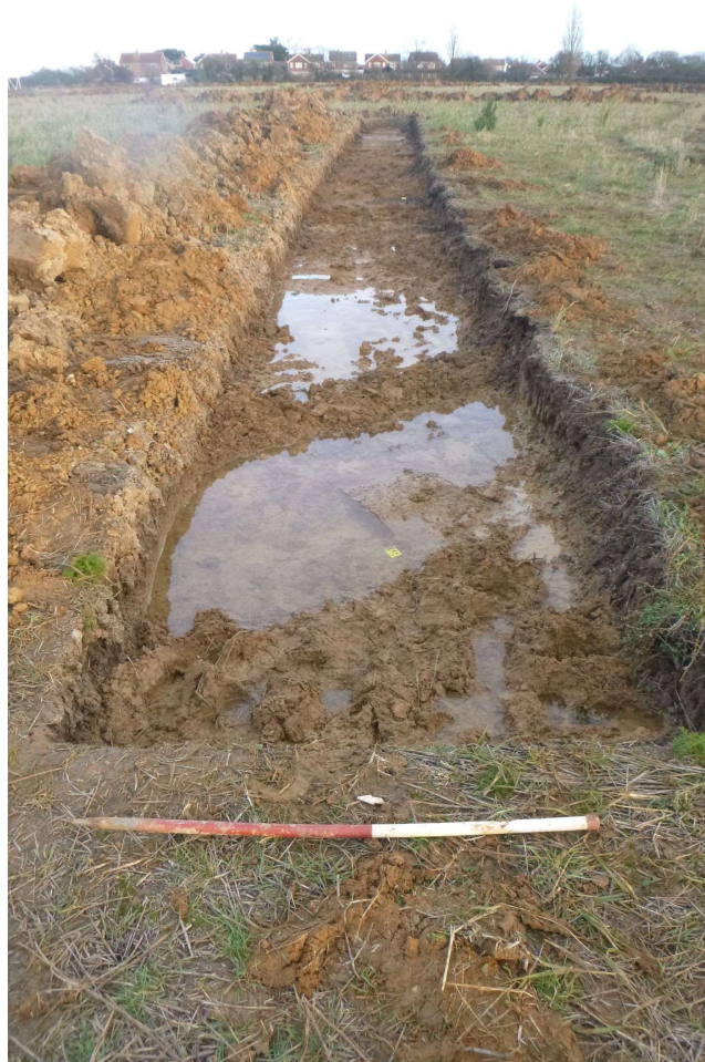
Photograph 7 T41 trench shot – looking east
