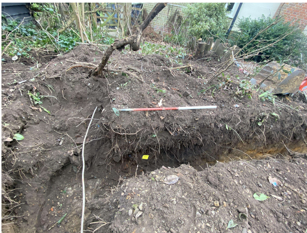
Photograph 3 SE edge of F1, looking roughly south.
