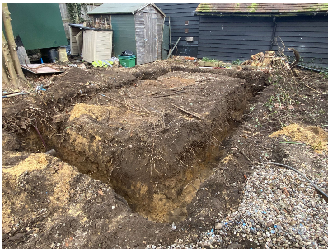
Photograph 1 General view of footings from SW corner, looking SE.
