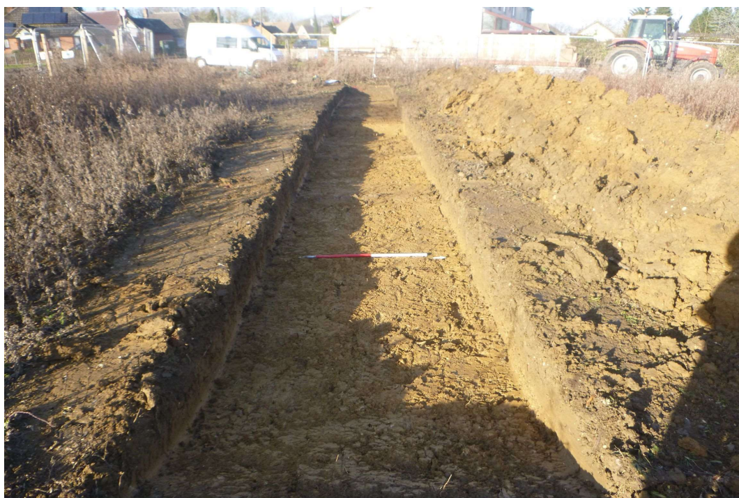
Photograph 5 T5 trench shot, looking west.
