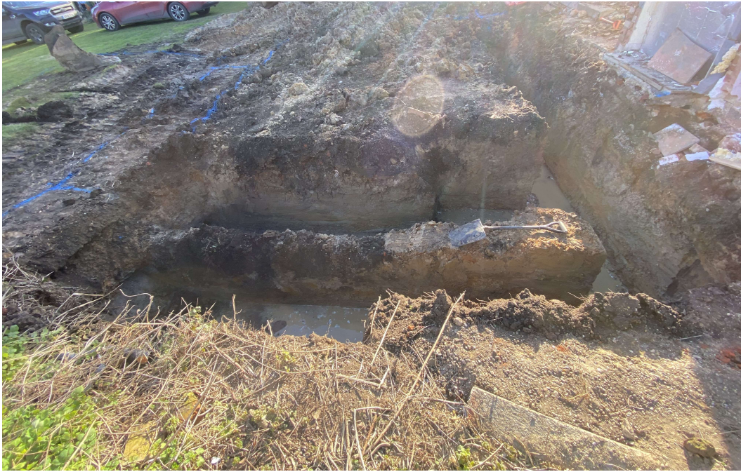
Photograph 2 West corner of footings, looking east.
