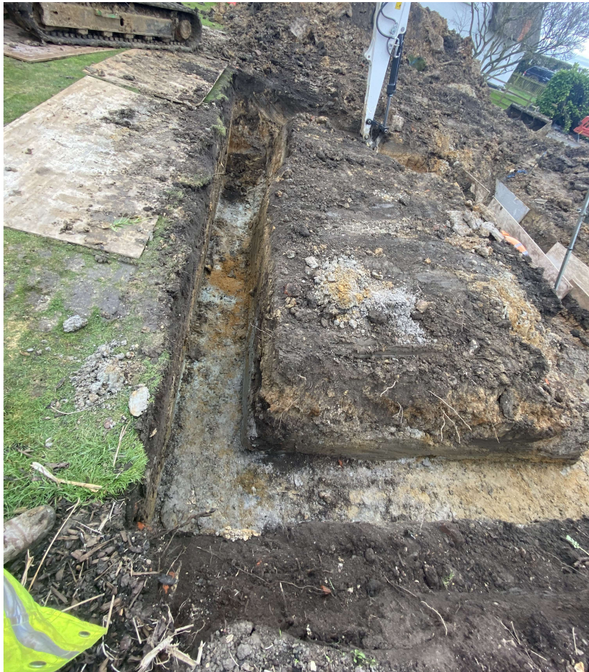
Photograph 3 View from north corner of site, looking SE.
