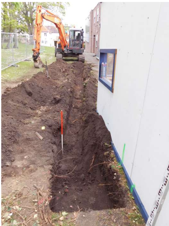
Photograph 36 Drainage trench west side of theatre, looking north.
