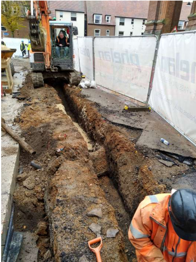
Photograph 35 Electricity cable trench, looking north.
