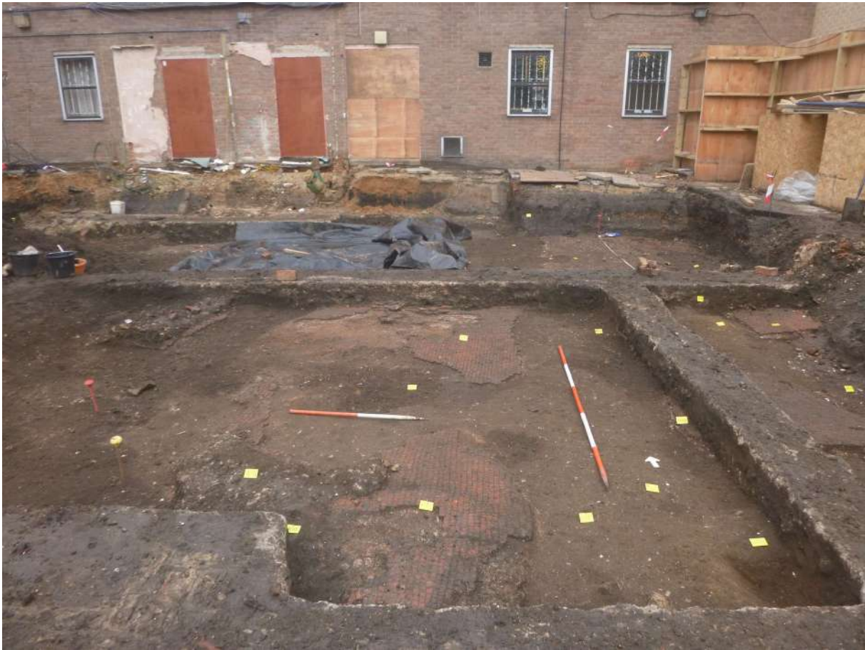
Photograph 9 Mercury House foundations cutting through Room C (centre, north/south aspect), Room F (far left), Room G (top right-hand corner) and Room I (right) of the Roman town-house, looking north. Post-Roman pits can also be seen to the right of the Room C tessellated floor.
