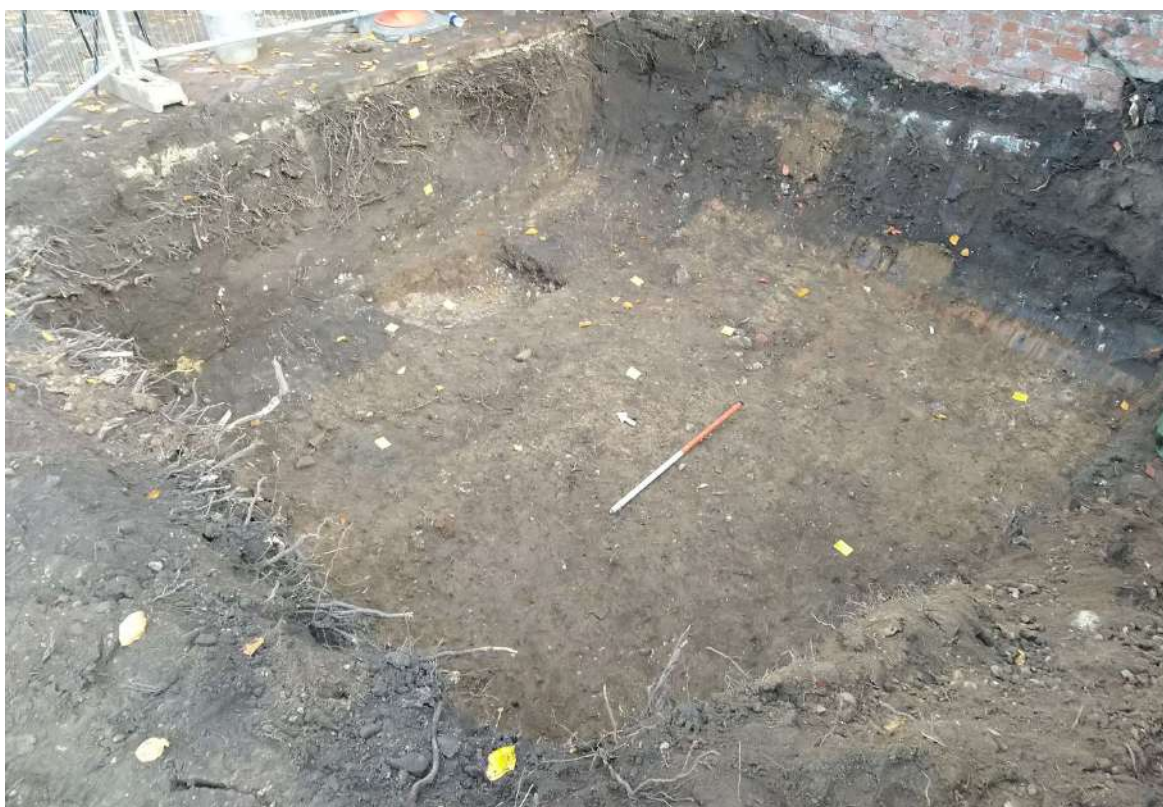
Photograph 33 Excavation of the footprint for the electricity sub-station, looking north-east.
