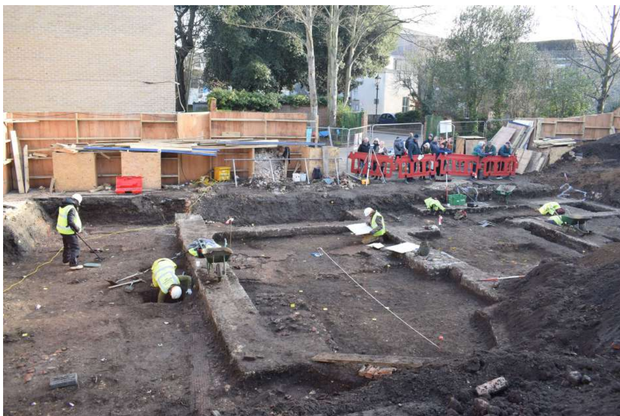
Photograph 2 The modern foundations of Mercury House cutting through Roman remains including the tessellated floor of Room C, looking east.
