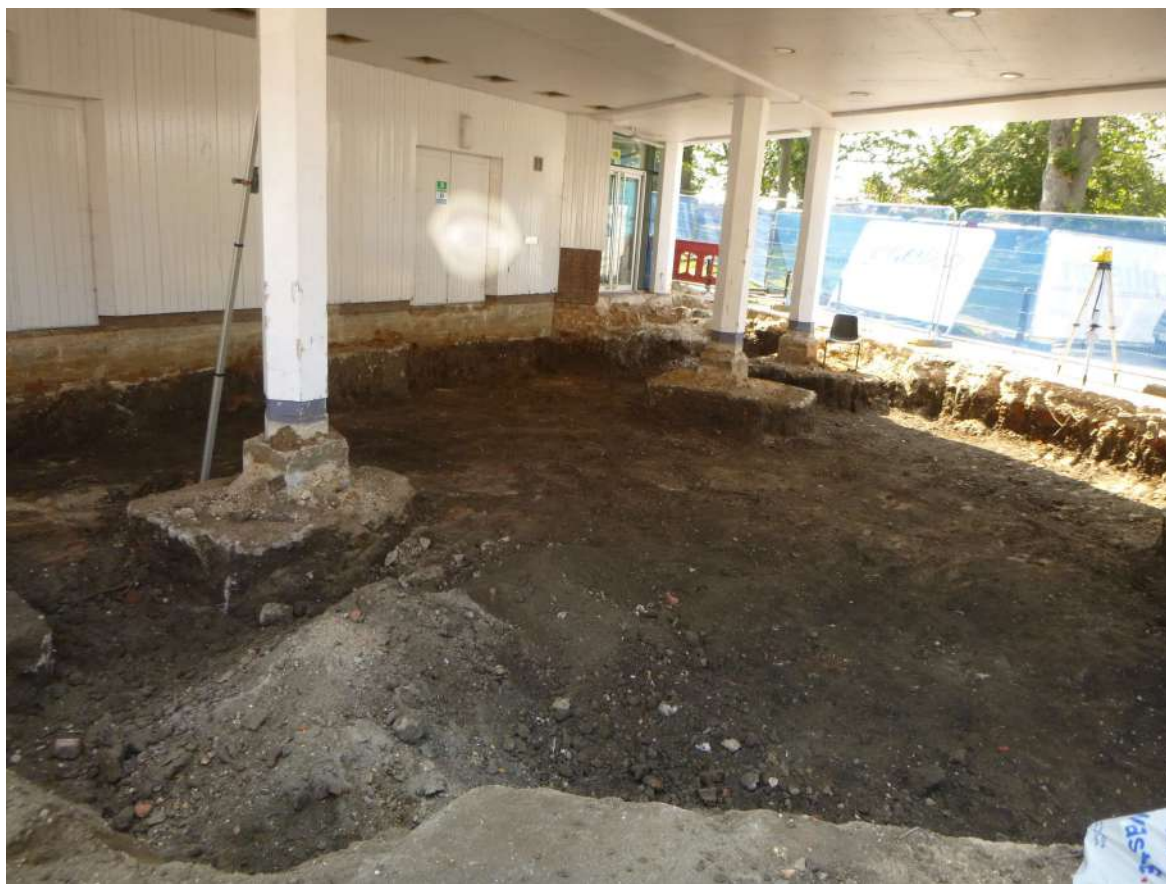
Photograph 32 Area C ground reduction, looking south-west.
