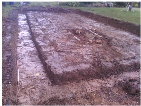
Photograph 2 Completed foundation trenching with inspection pit - view south
