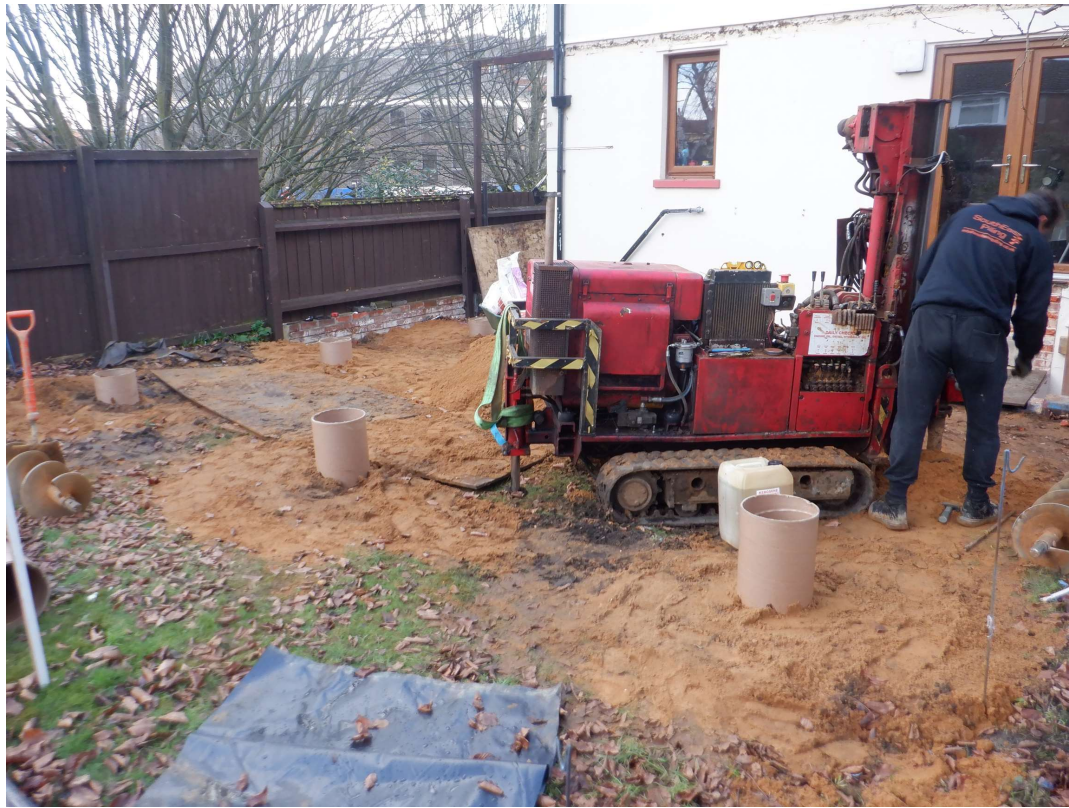
Photograph 2 Site shot – view north-east
