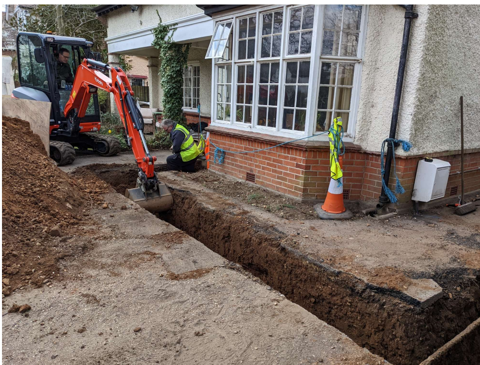
Photograph 3 Site shot, looking south-west
