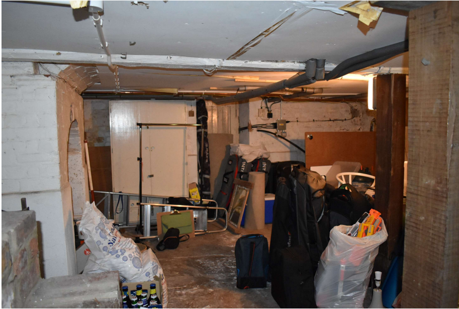
Photograph 1 Interior of cellar. Photograph taken facing east.
