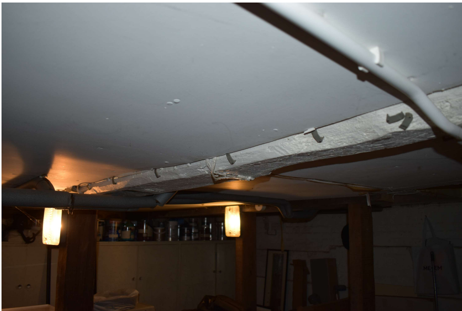
Photograph 6 Detail of original bridging beam. Photograph taken facing south-west.
