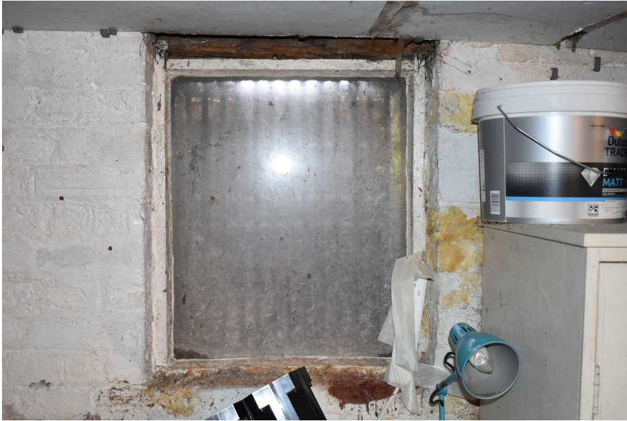
Photograph 5 Detail of window. Photograph taken facing south.
