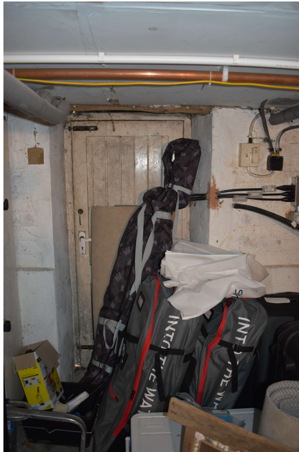
Photograph 7 Detail of eastern door. Photograph taken facing east.
