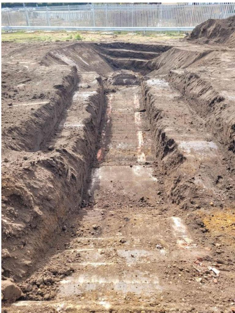
**Photograph 2** Looking down into turntable pit, showing staircase, external concrete ring, brick walls and central pivot, looking south-west
