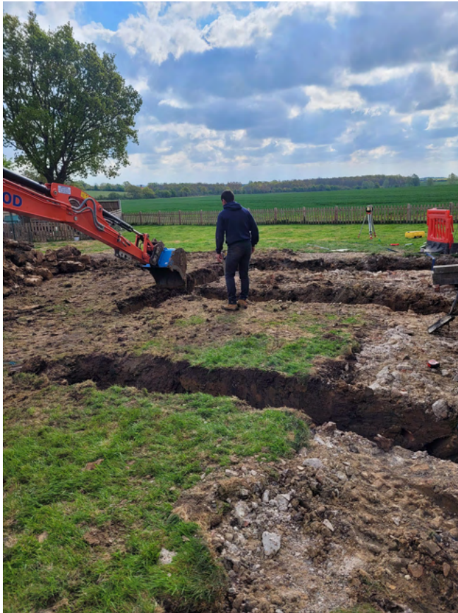
Photograph 4 General shot of extension foundations, looking east-south-east
