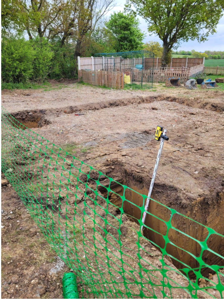
Photograph 5 General site shot of garage foundations, facing east-north-east
