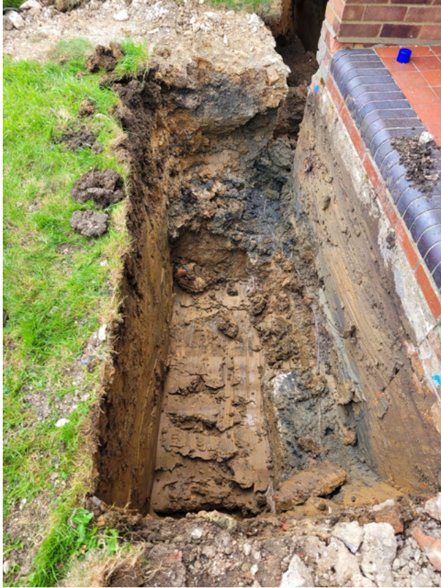
Photograph 3 Porch excavation area, looking north-east
