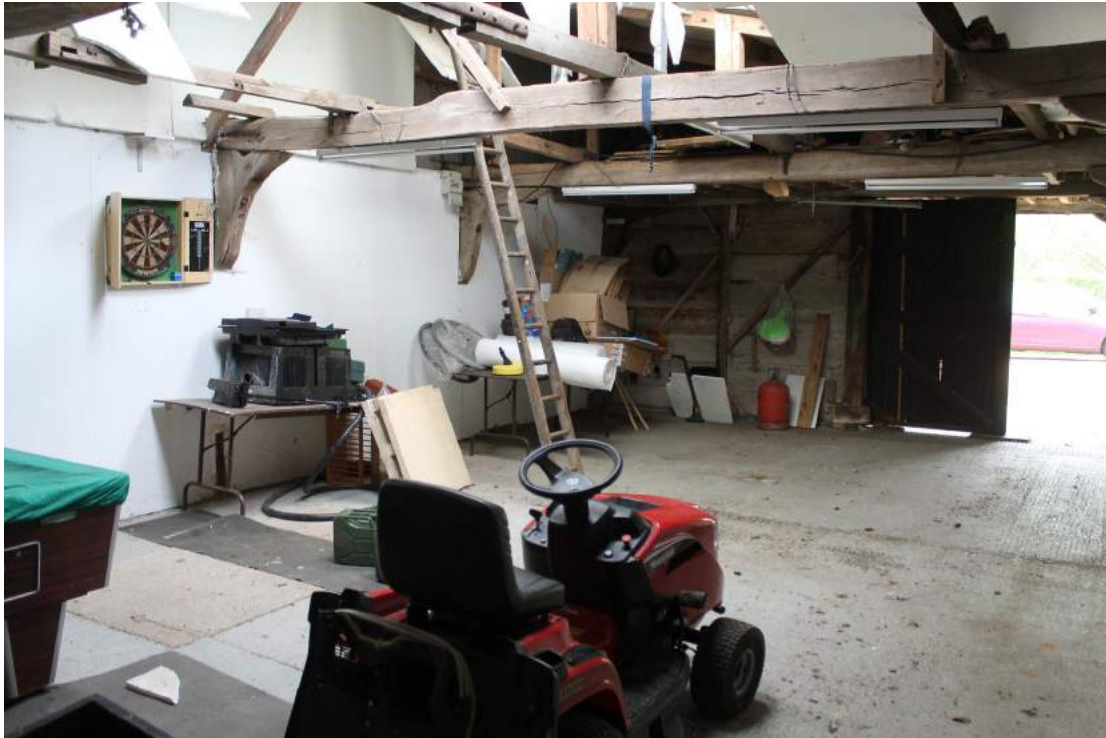
Photograph 13 Inserted loft above bays B4 and B5, accessible only by ladder – view north-east.
