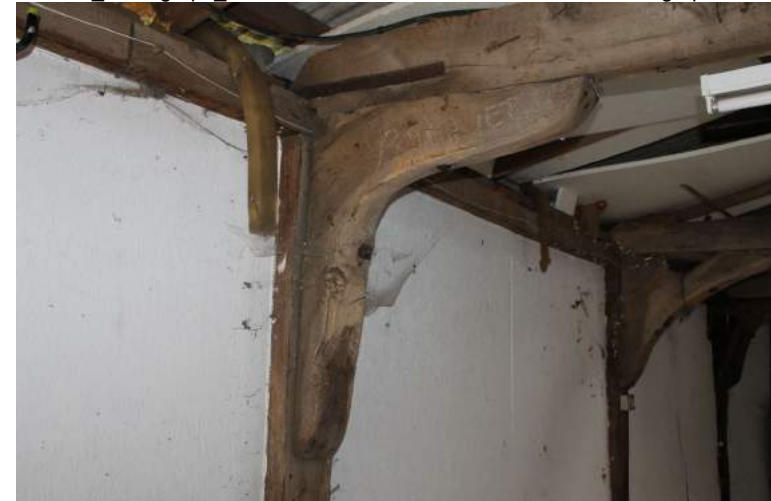
CGPF22_Photograph_023Southern knee-brace of tie-beam 2. Photograph take... CGPF22_Photograph_024Northern knee-brace of tie-beam 3. Photograph take...
