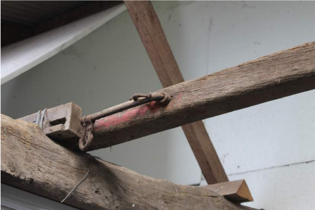
Photograph 16 Waggon shaft (complete with harness attachment) fixed to a section of door post to form a crude longitudinal purlin supporting the struts of the modern roof.
