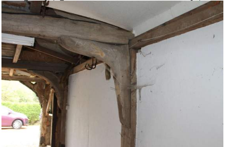
CGPF22_Photograph_023Southern knee-brace of tie-beam 2. Photograph take... CGPF22_Photograph_024Northern knee-brace of tie-beam 3. Photograph take...
