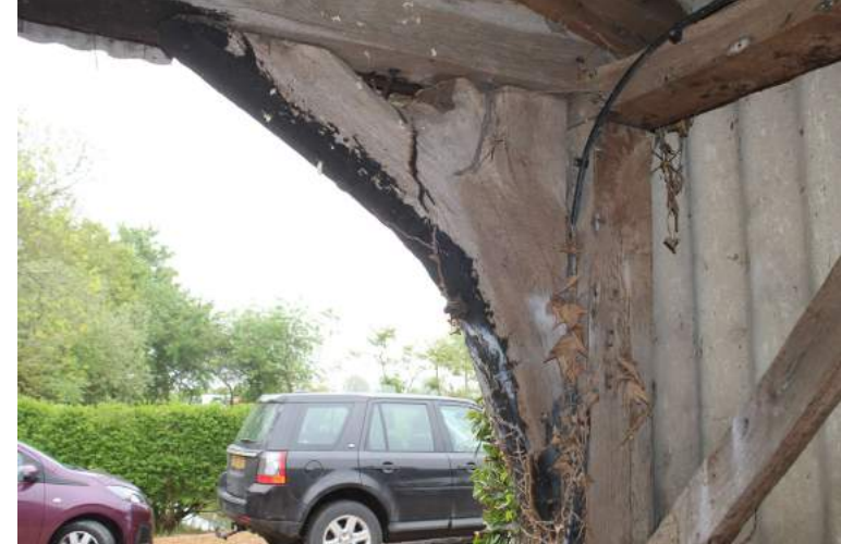
CGPF22_Photograph_031Southern knee-brace of tie-beam 5. Photograph take...
