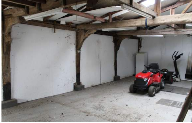
CGPF22_Photograph_012Northern knee-brace of tie-beam 1. Photograph take...
