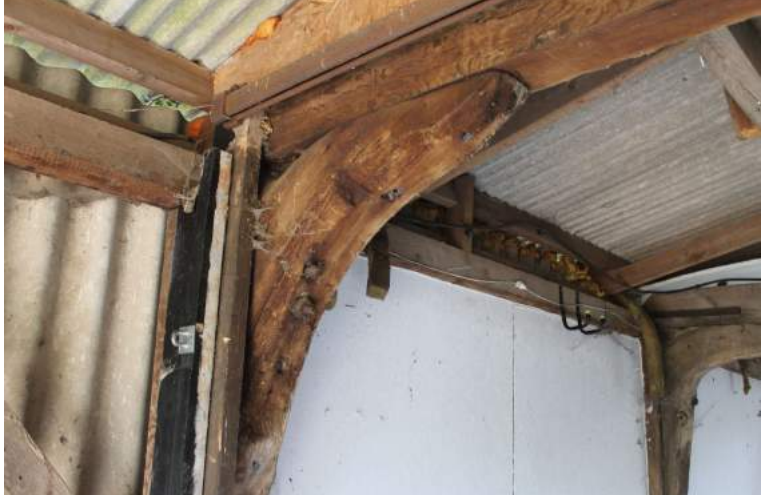
CGPF22_Photograph_030Southern knee-brace of tie-beam 5. Photograph take...
