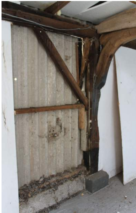
Photograph 6 Inserted frame to the cart lodge openings on the south wall.
