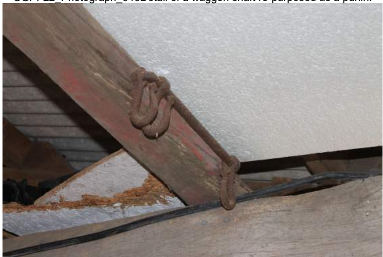
CGPF22_PhotoGraph_046Detail of a waggon shaft re-purposed as a purlin.
