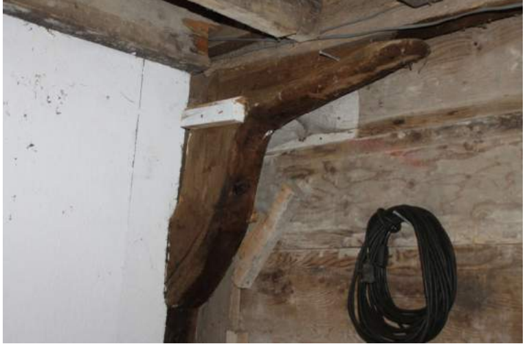
CGPF22_Photograph_028Southern knee-brace of tie-beam 4. Photograph take...
