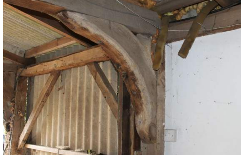
CGPF22_Photograph_029Northern knee-brace of tie-beam 5 (exterior). Photog...
