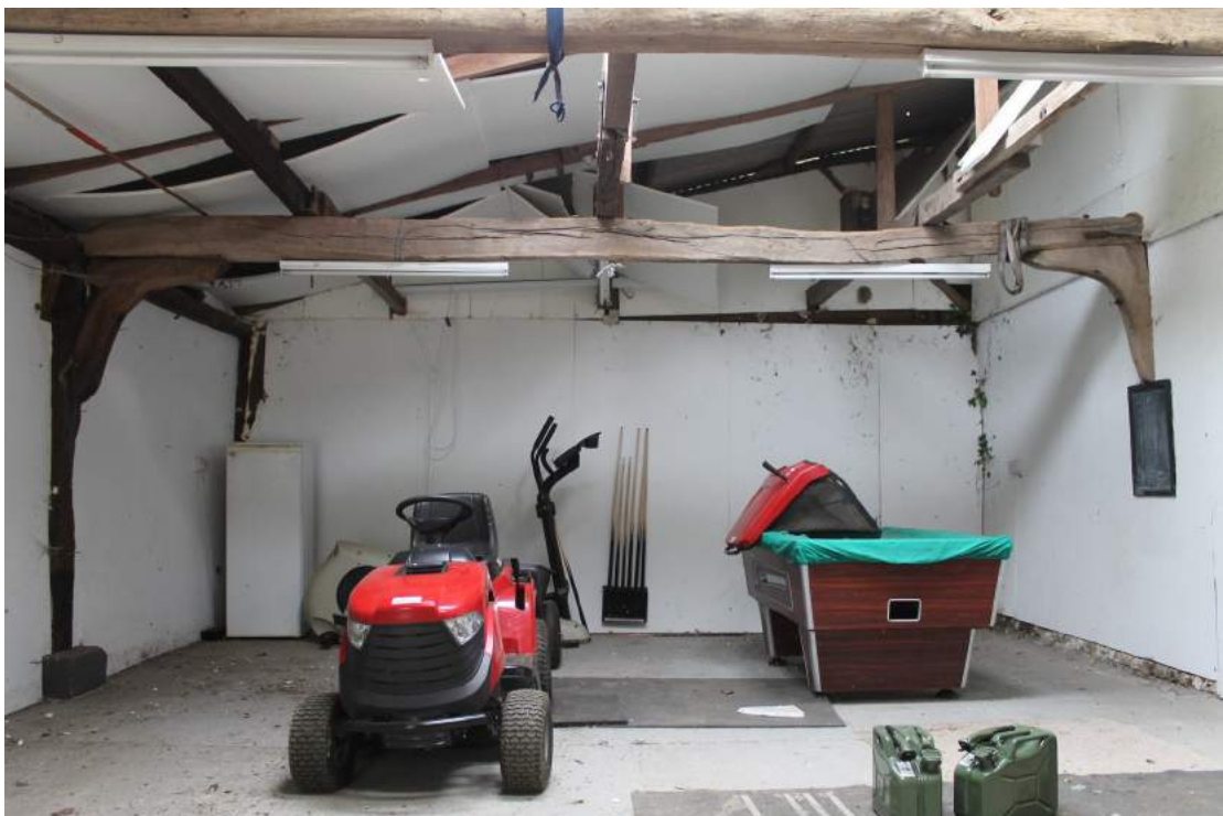
Photograph 10 Tie-beam T1 with knee braces – view west.
