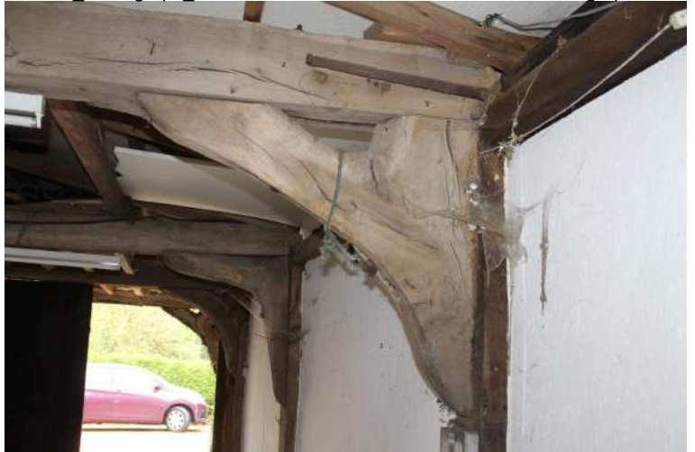
CGPF22_Photograph_021Northern knee-brace of tie-beam 3. Photograph take... CGPF22_Photograph_022Northern knee-brace of tie-beam 3. Photograph take...
