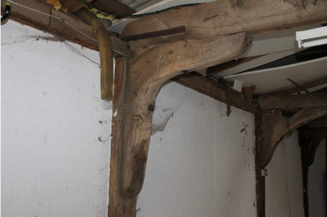
Photograph 11 Knee brace at south end of tie-beam T3 showing iron bolts to the post and tie-beam and the iron staple at the end of the tie-beam – view south-west.
