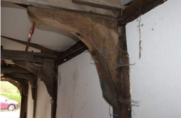
CGPF22_Photograph_015Southern knee-brace of tie-beam 1. Photograph take...
