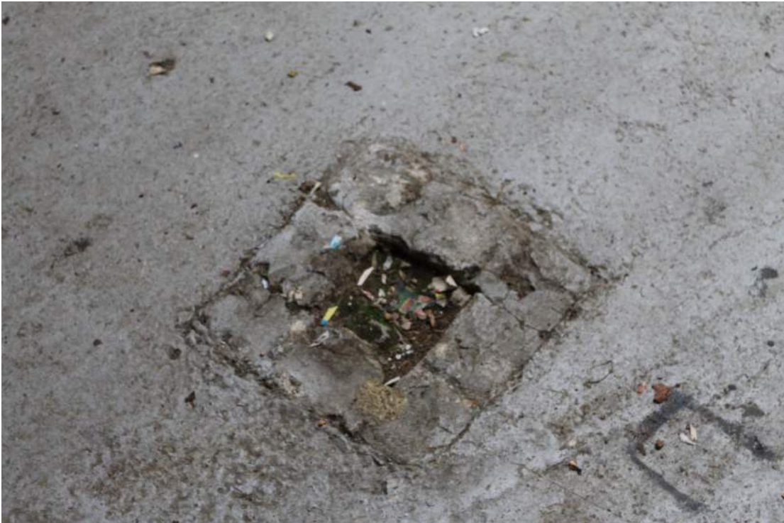
Photograph 14 Scar in the concrete floor from the removal of the inserted post below tie-beam T3, which provided support for the loft.
