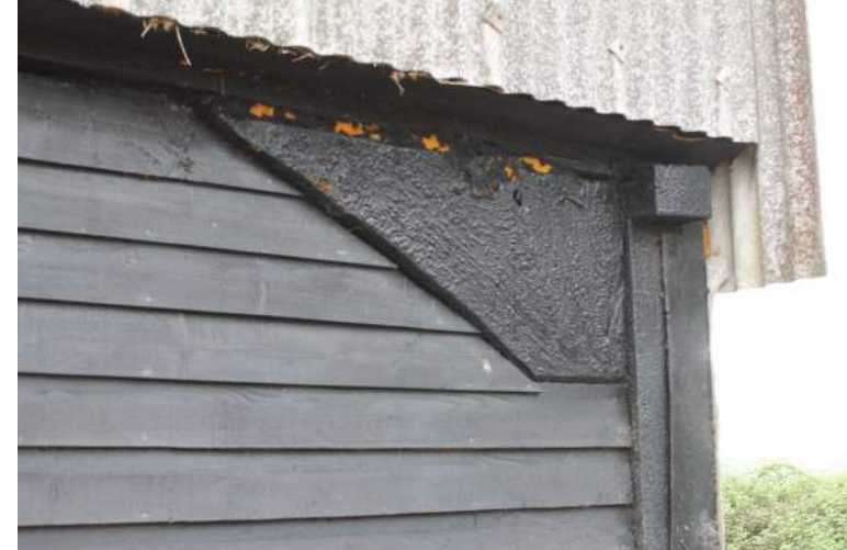
CGPF22_Photograph_031Southern knee-brace of tie-beam 5. Photograph take...
