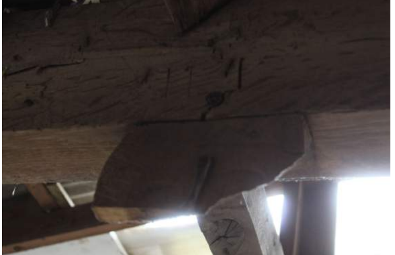
CGPF22_Photograph_038Foot of inserted post supporting tie-beam 4 resting o...
