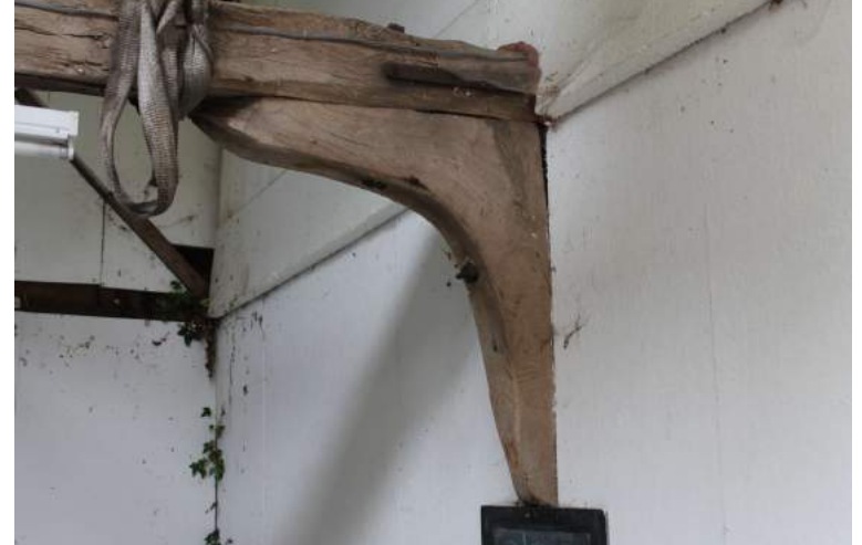
CGPF22_Photograph_014Southern knee-brace of tie-beam 1. Photograph take...
