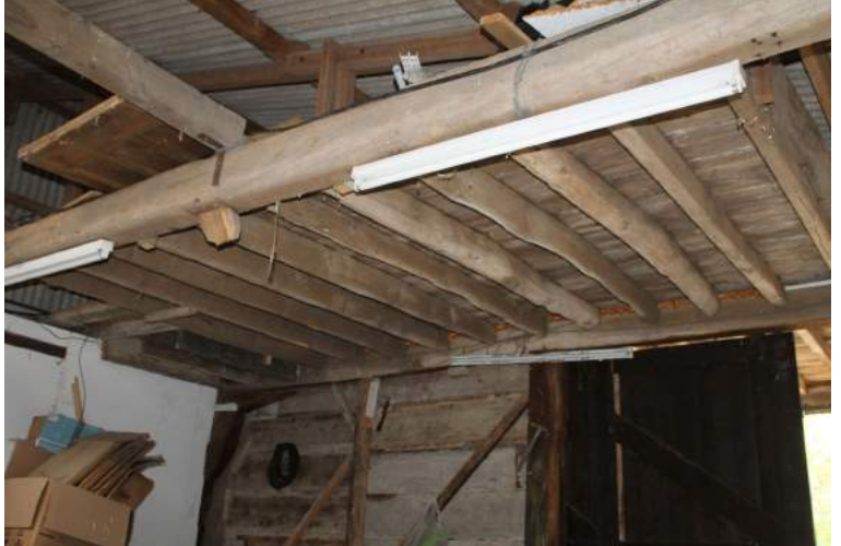
CGPF22_Photograph_032Inserted loft above bays 4 and 5. Photograph taken f...
