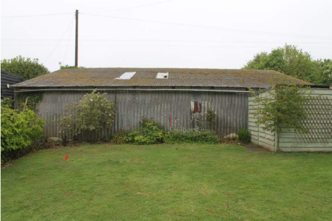
Photograph 2 South elevation – view north.
