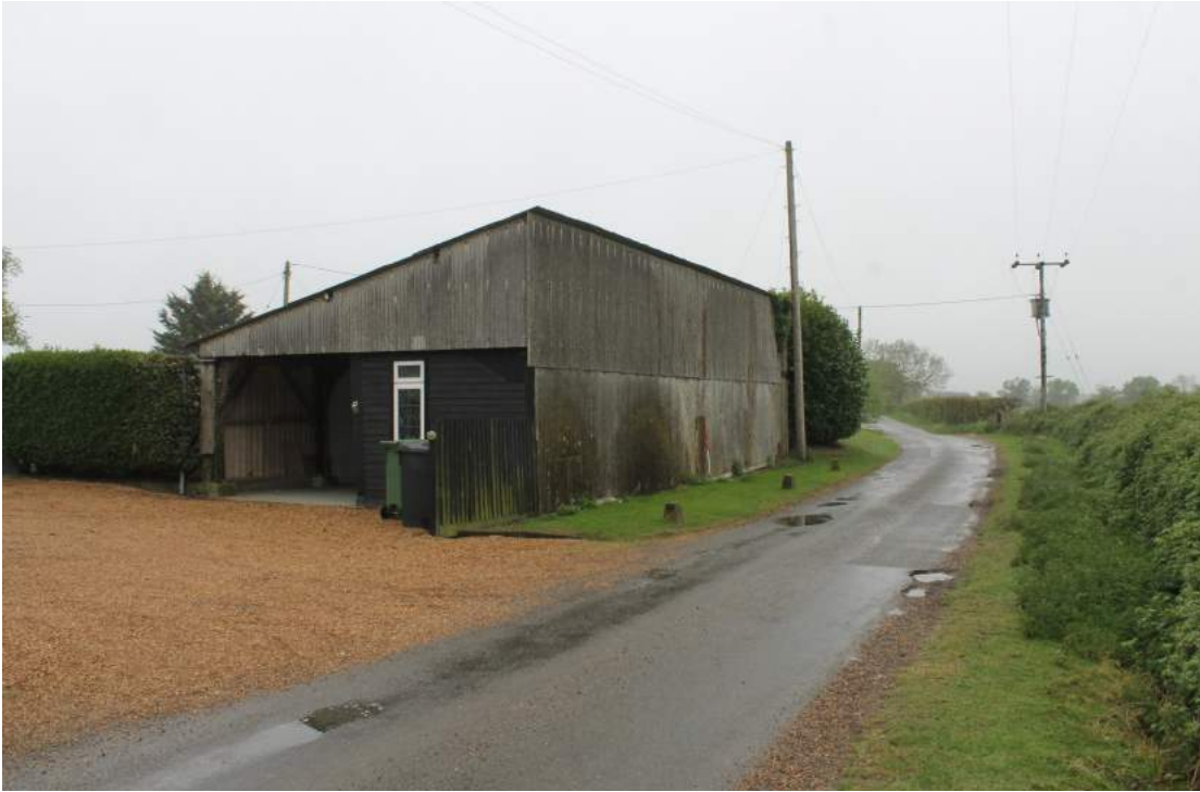
Photograph 1 North and east elevations – view south-west.
