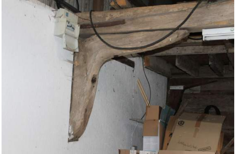
CGPF22_Photograph_023Southern knee-brace of tie-beam 2. Photograph take... CGPF22_Photograph_024Northern knee-brace of tie-beam 3. Photograph take...
