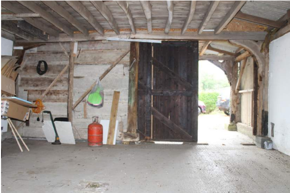
Photograph 9 Inserted dividing wall between bays B4 and B5 with the loft above.
