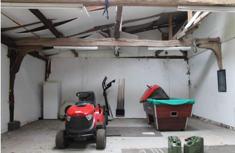
CGPF22_Photograph_013Northern knee-brace of tie-beam 1. Photograph take...
