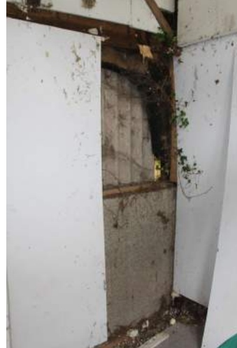
CGPF22_PhotoGraph_046Detail of a waggon shaft re-purposed as a purlin.
