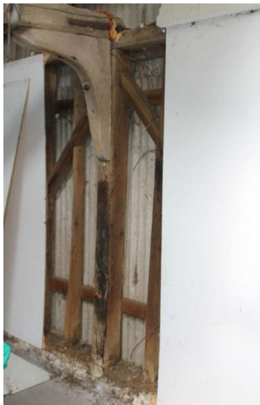
Photograph 5 Exposed timber-frame of the north wall.
