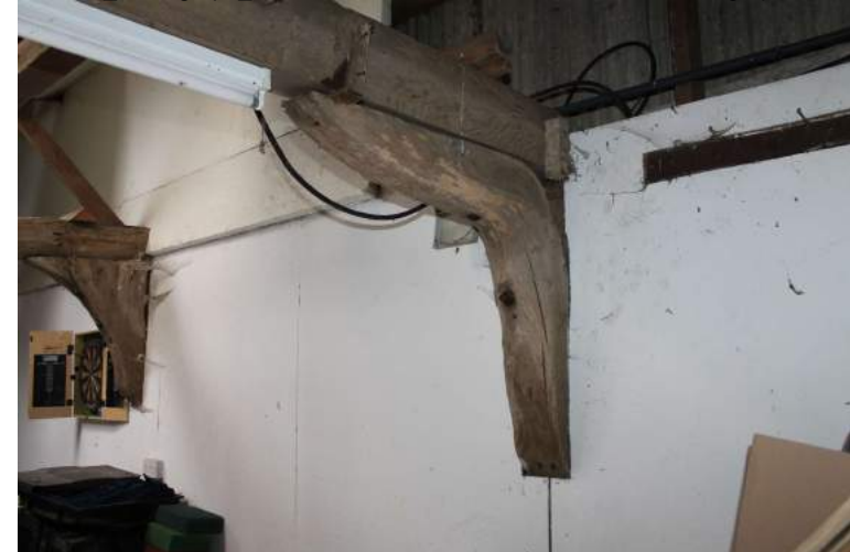
CGPF22_Photograph_023Southern knee-brace of tie-beam 2. Photograph take... CGPF22_Photograph_024Northern knee-brace of tie-beam 3. Photograph take...
