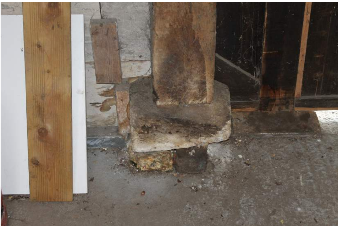
Photograph 15 Inserted post below tie-beam T4 providing support for the loft, with a timber pillow carried on bricks – view east.
