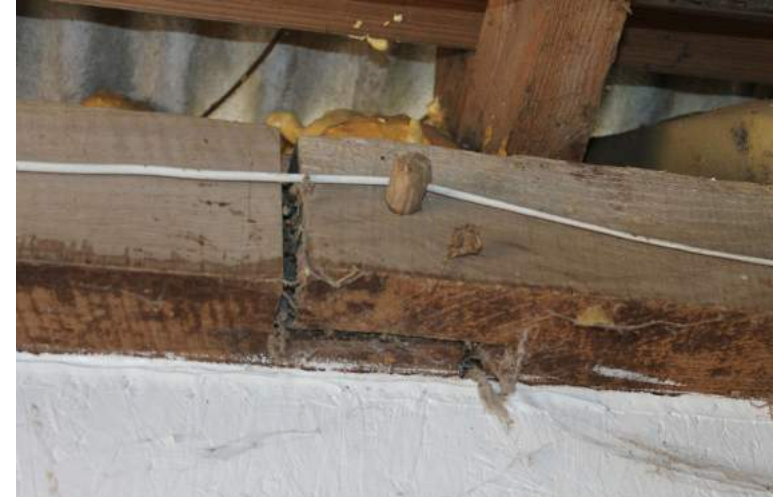
CGPF22_Photograph_039Wall plate face-halved and timber-pegged scarf joint.
