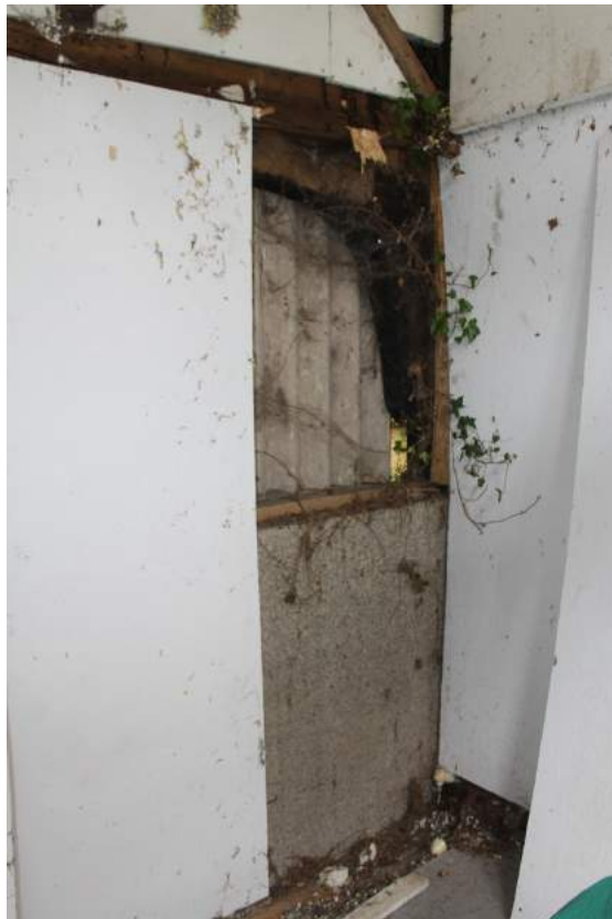
Photograph 8 Inserted breeze block wall to west end of the cart lodge.
