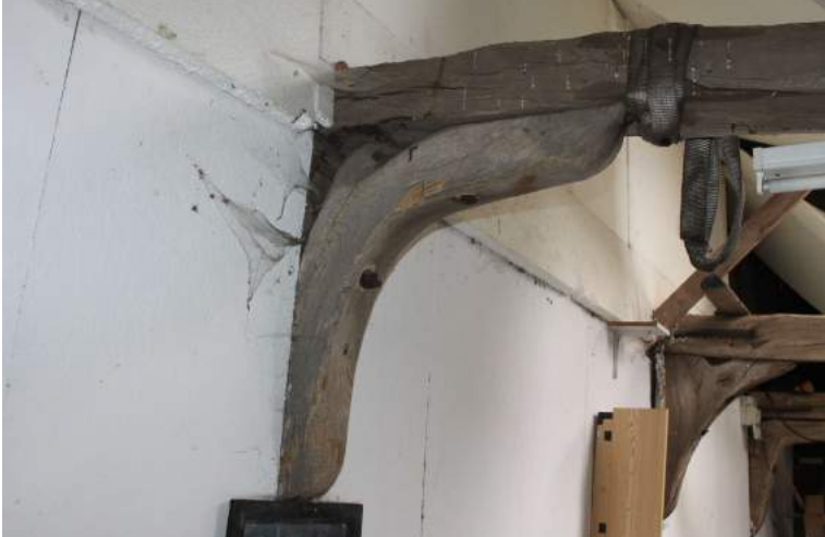
CGPF22_Photograph_015Southern knee-brace of tie-beam 1. Photograph take...
