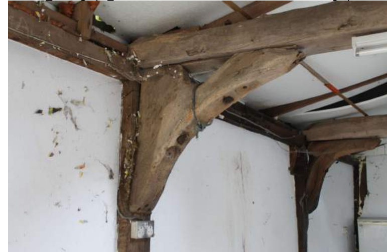
CGPF22_Photograph_021Northern knee-brace of tie-beam 3. Photograph take... CGPF22_Photograph_022Northern knee-brace of tie-beam 3. Photograph take...
