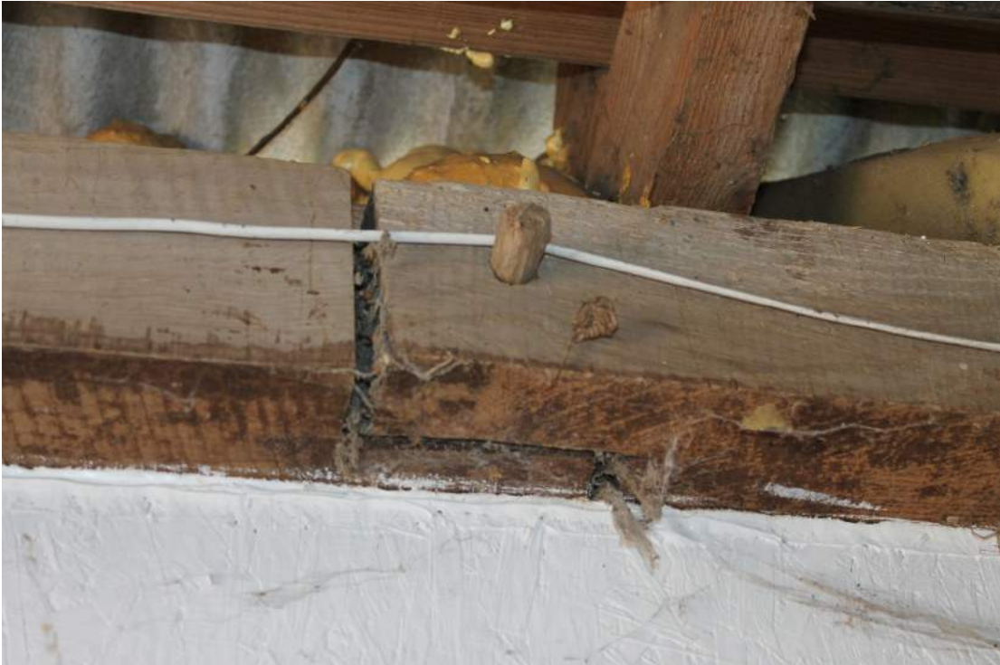
Photograph 7 Face-halved and single-pegged scarf joint in the wall plate of the south wall.
