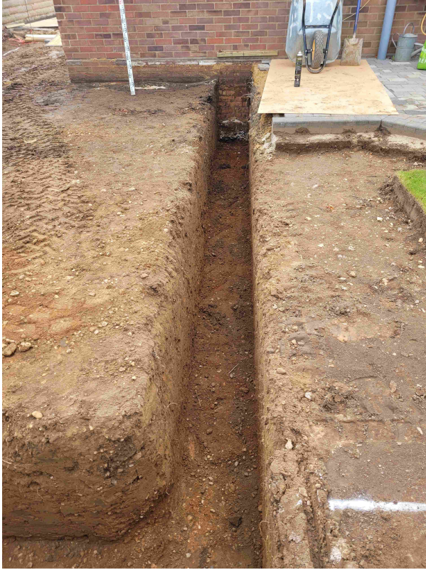
Photograph 3 Trench shot, looking south-east
