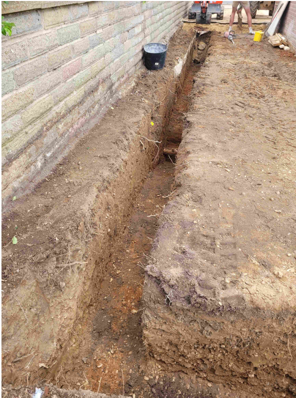
Photograph 4 Trench shot, looking south-east
