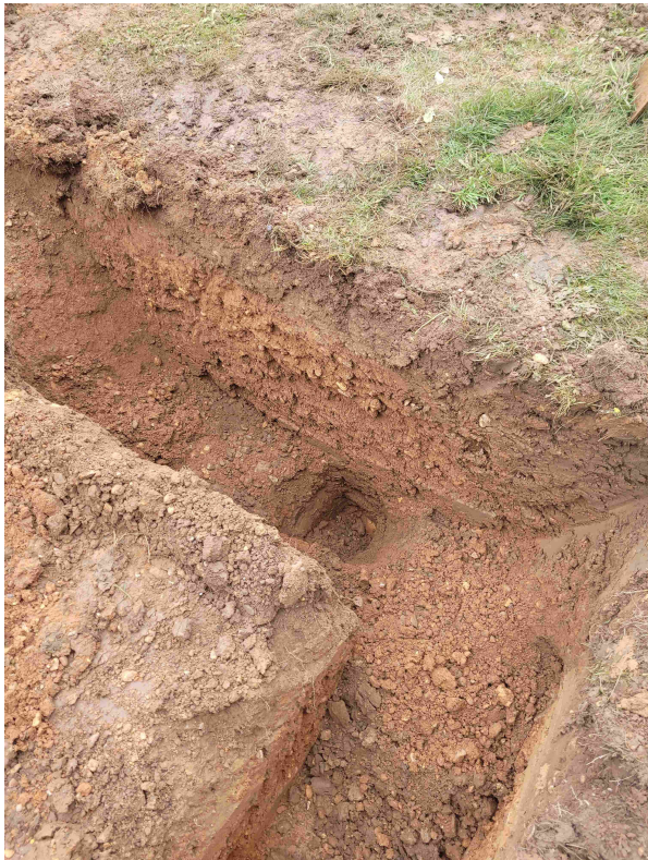
Photograph 3 Trench shot showing water pipe discovered in the south-eastern corner
