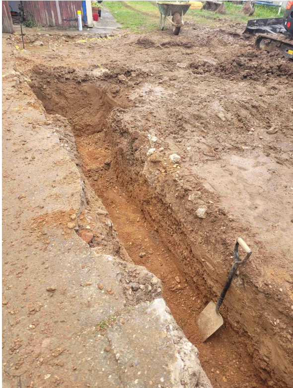
Photograph 2 Trench shot, looking north-east
