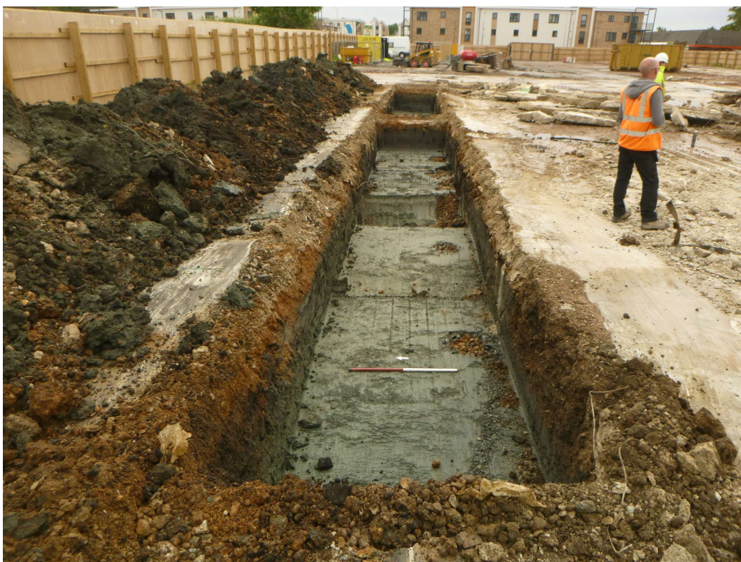
Photograph 3 T4 trench shot – view east.
