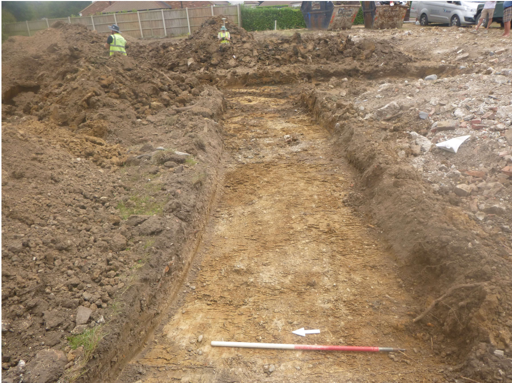
Photograph 1 Trench 1, view east
