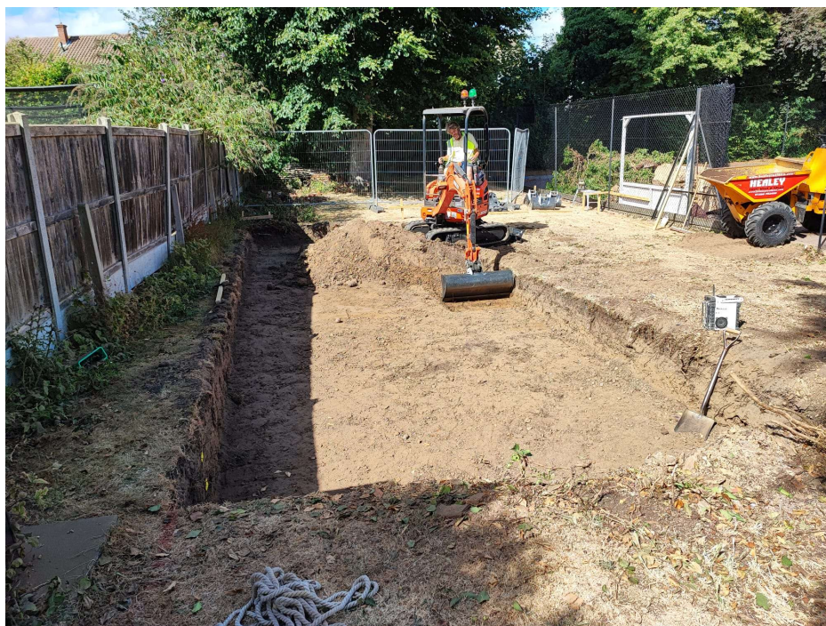
Photograph 1 Pad 1, looking north-east
