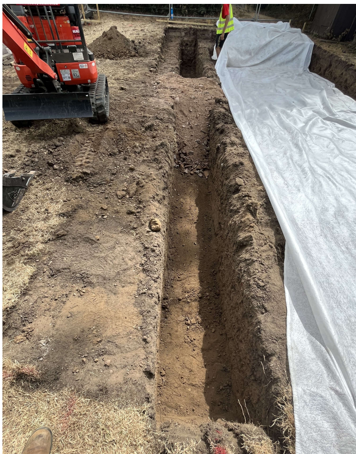
Photograph 3 Excavation of drainage trench, looking north
