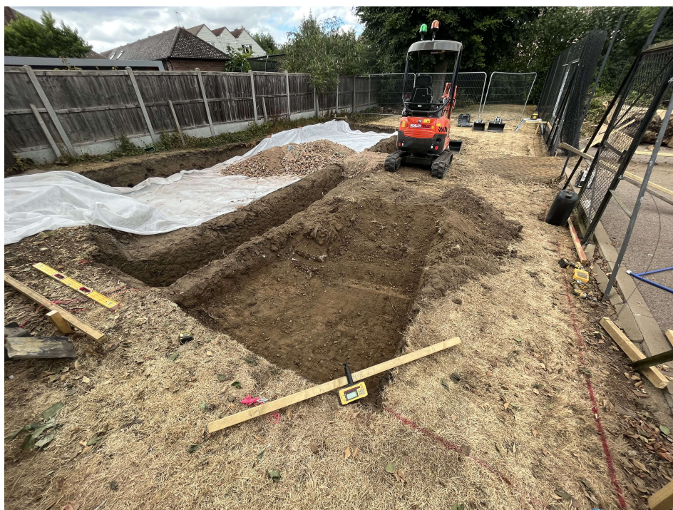
Photograph 2 Excavation of Pad 2, looking north-west
