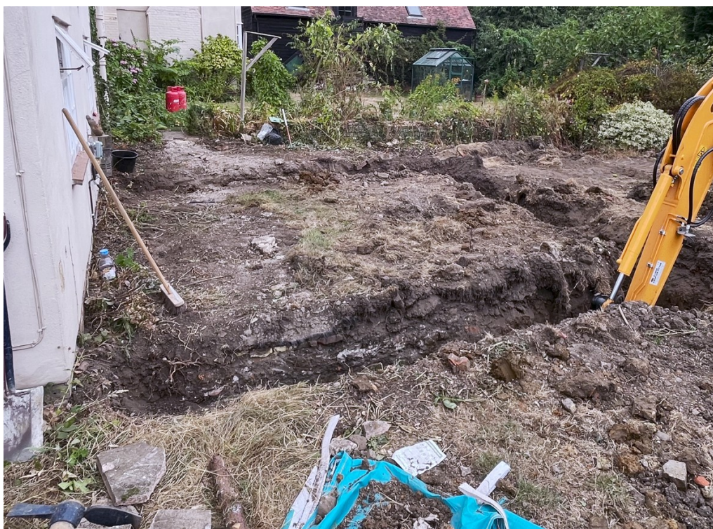
Photograph 4 General view of foundation trench from eastern side, looking west.
