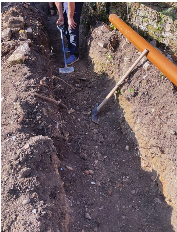
Photograph 5 Western edge of the drainage trench, looking south.
