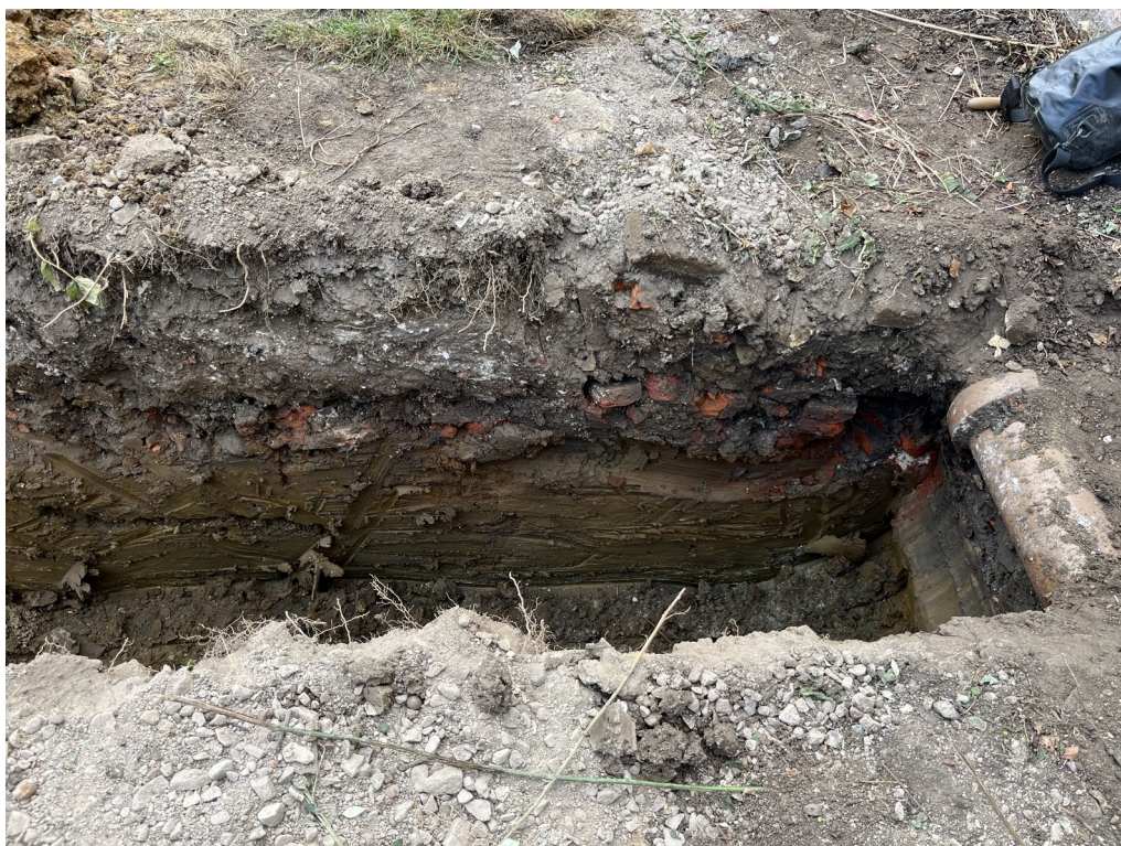
Photograph 3 Western edge of main foundation trench, looking east.
