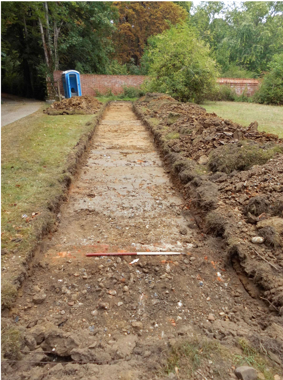
Photograph 1 Trench 1 showing brick wall foundation F3 in the foreground, looking north-north-west.
