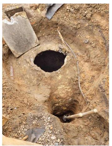
Photograph 8 Partially exposed top of well showing brick outer edges and services
