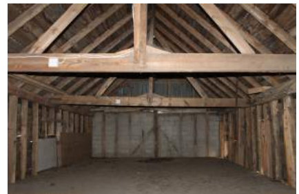
MHGF22_PhotoGraph33Upper floor and roof view (facing SE)
