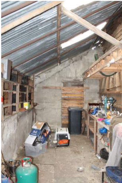
MHGF22_PhotoGraph17Lean-to at rear of building
