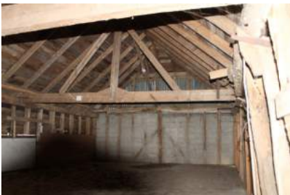
MHGF22_PhotoGraph25Roof and mezzanine (facing SE)
