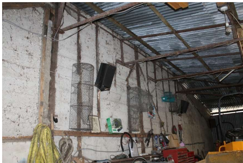
Photograph 9 Extension B – view north-east
