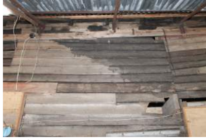
MHGF22_Photo38Weatherboarding on internal wall NW wall
