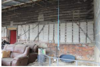
MHGF22_PhotoGraph20North-east side, inside covered area
