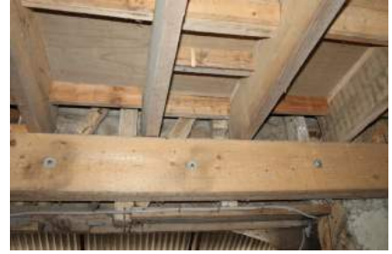
MHGF22_PhotoGraph03Detail of new floor over old timbers
