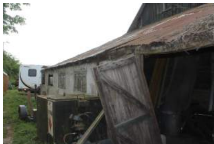
MHGF22_PhotoGraph05External SE wall
