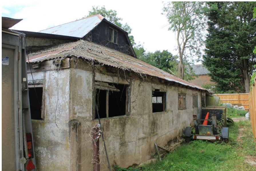
Photograph 4 Extension C – view south-west
