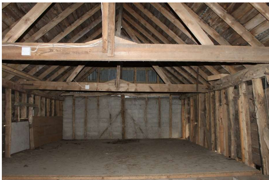
Photograph 13 The inserted mezzanine of the barn - view south-east
