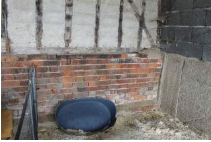
MHGF22_PhotoGraph01Brick plinth and downward wall (north-east side)
