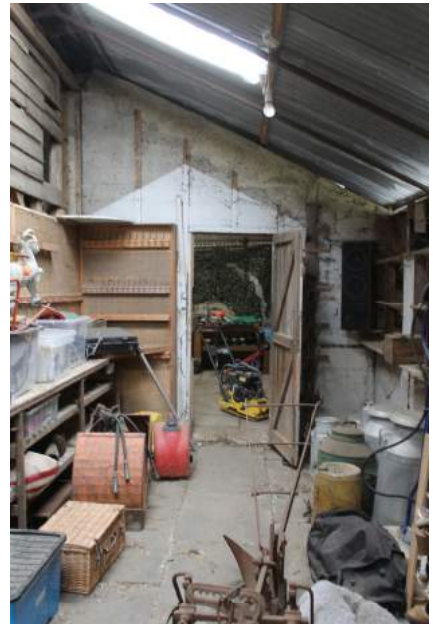
MHGF22_PhotoGraph18Lean-to at rear of building (facing SW)
