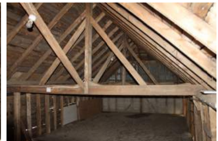
MHGF22_PhotoGraph26Roof and mezzanine facing SE
