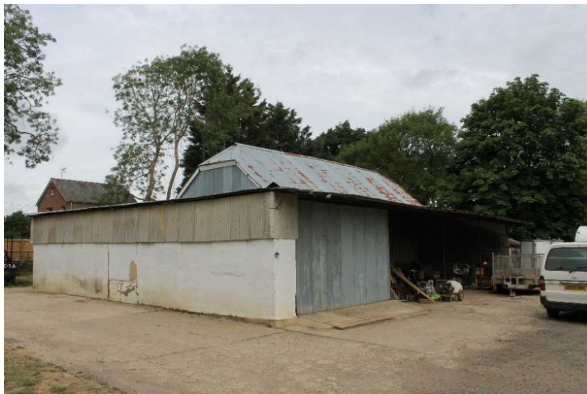
Photograph 2 The south-east elevation showing extension B – view west
