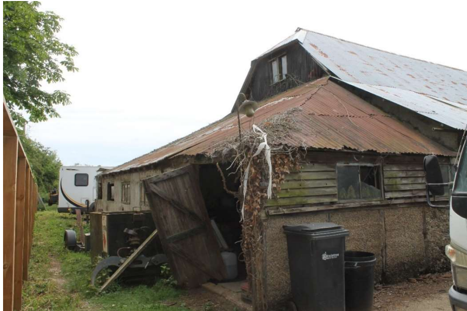
Photograph 3 Extension C on the north-west elevation – view east
