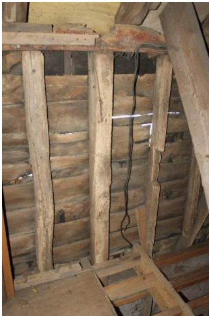
MHGF22_PhotoGraph32Timber frame detail
