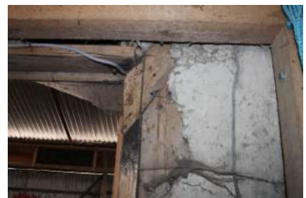
MHGF22_PhotoGraph36Wall and doorway detail
