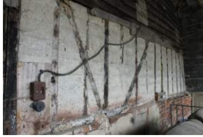
MHGF22_PhotoGraph02Concrete filled timber wall (NE side)
