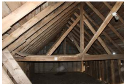
MHGF22_PhotoGraph27Roof and mezzanine facing SE
