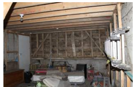
MHGF22_PhotoGraph09Ground floor facing NW
