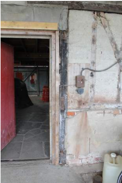
MHGF22_PhotoGraph04Doorway in north-east wall
