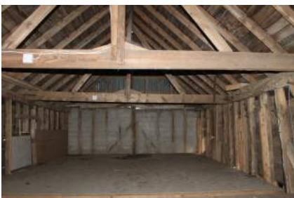
MHGF22_PhotoGraph34Upper floor timber frame
