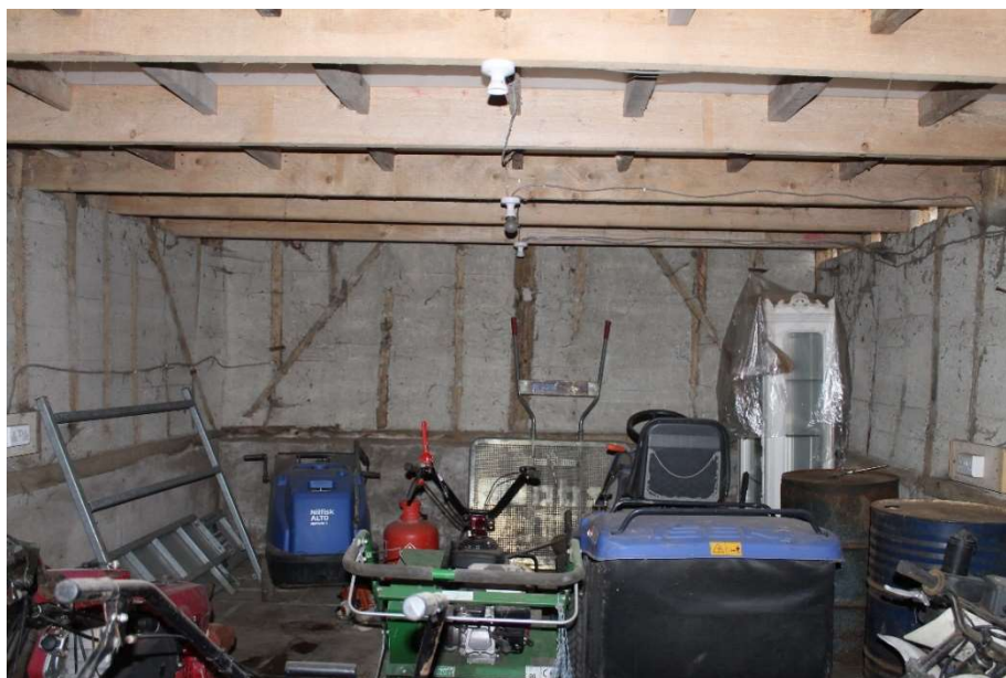
Photograph 11 The interior of the barn with the modern concrete infill between the posts of the frame - view south-east
