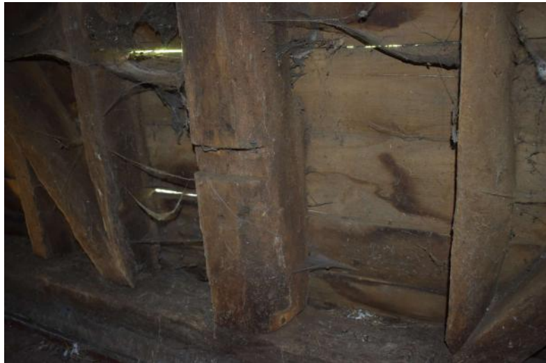
SOWBF22_PhotoGraph_059Detail of reused timber post in store 4. Ph... SOWBF22_PhotoGraph_060Detail of reused timber for sill-beam in stor...
