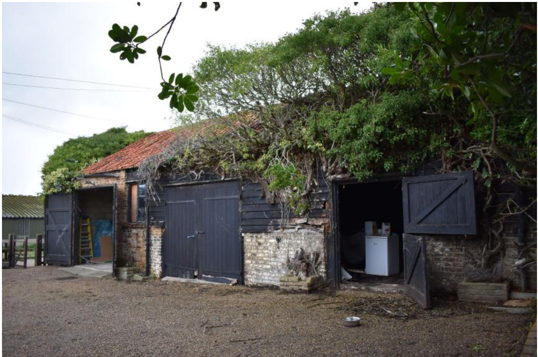
Photograph 1 South-east elevation. Photograph taken facing north north-west.
