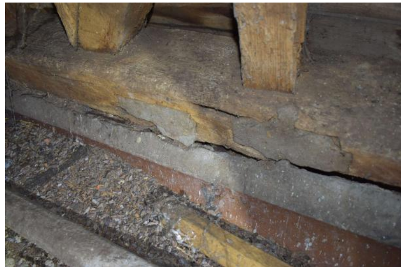
SOWBF22_PhotoGraph_065Detail of scarf joint in sill-beam in store 3. ... SOWBF22_PhotoGraph_066Detail of metal strap in tie-beam between ...
