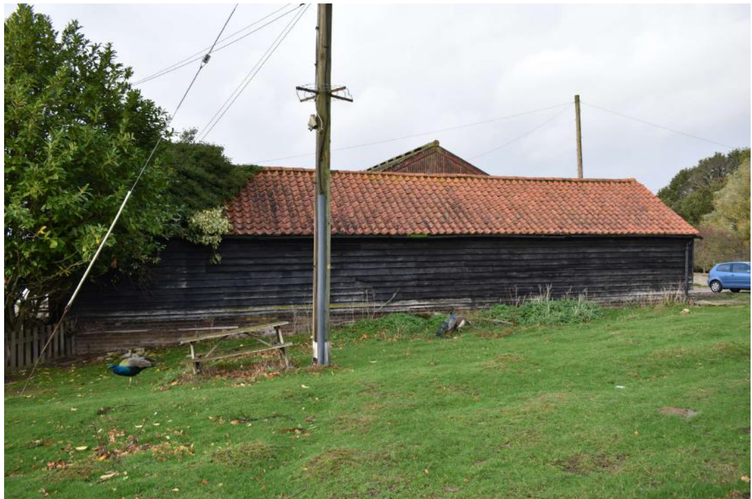
Photograph 5 North-east elevation. Photograph taken facing west.
