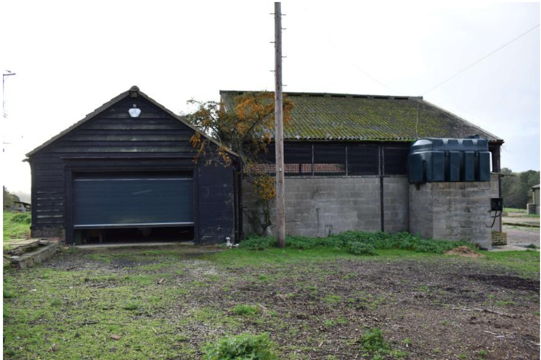
Photograph 4 North-west elevation. Photograph taken facing south-east.
