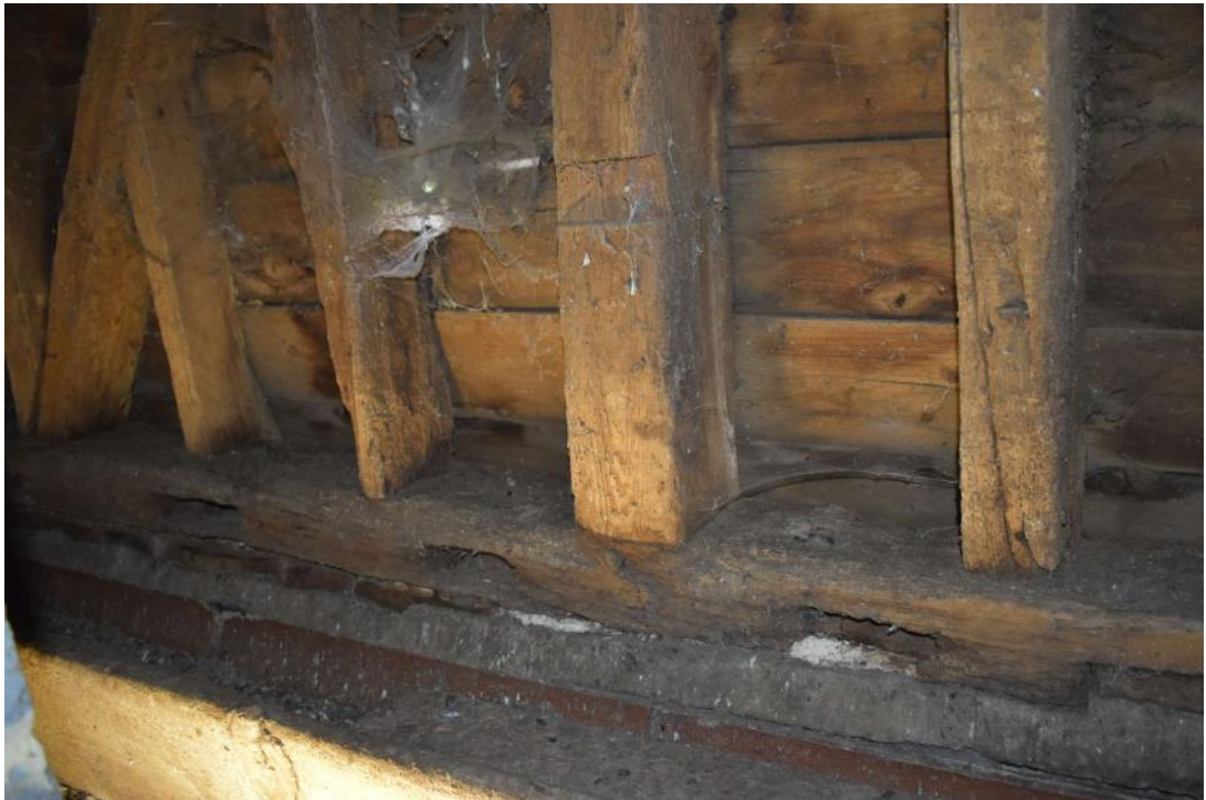
Photograph 14 Detail of reused timber for sill-beam in Store 4. Photograph taken facing north-east.
