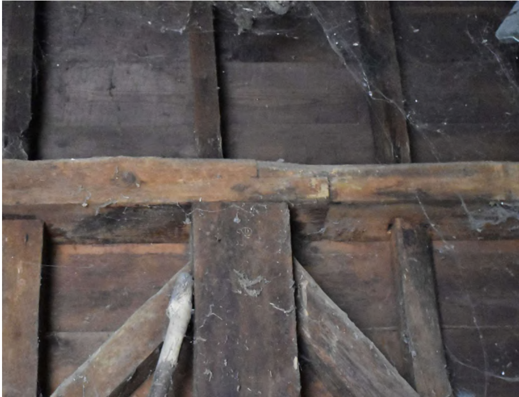
Photograph 15 Detail of scarf joint in wall plate of Store 3. Photograph taken facing north-west.
