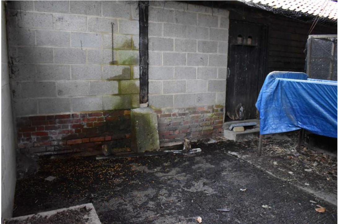
Photograph 8 Detail of original post and brick plinth in Store 5. Photograph taken facing south-east.
