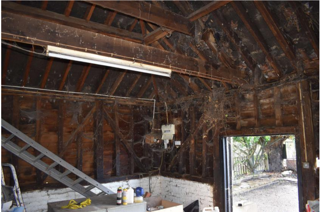
Photograph 11 Interior of Store 3. Photograph taken facing south-east.
