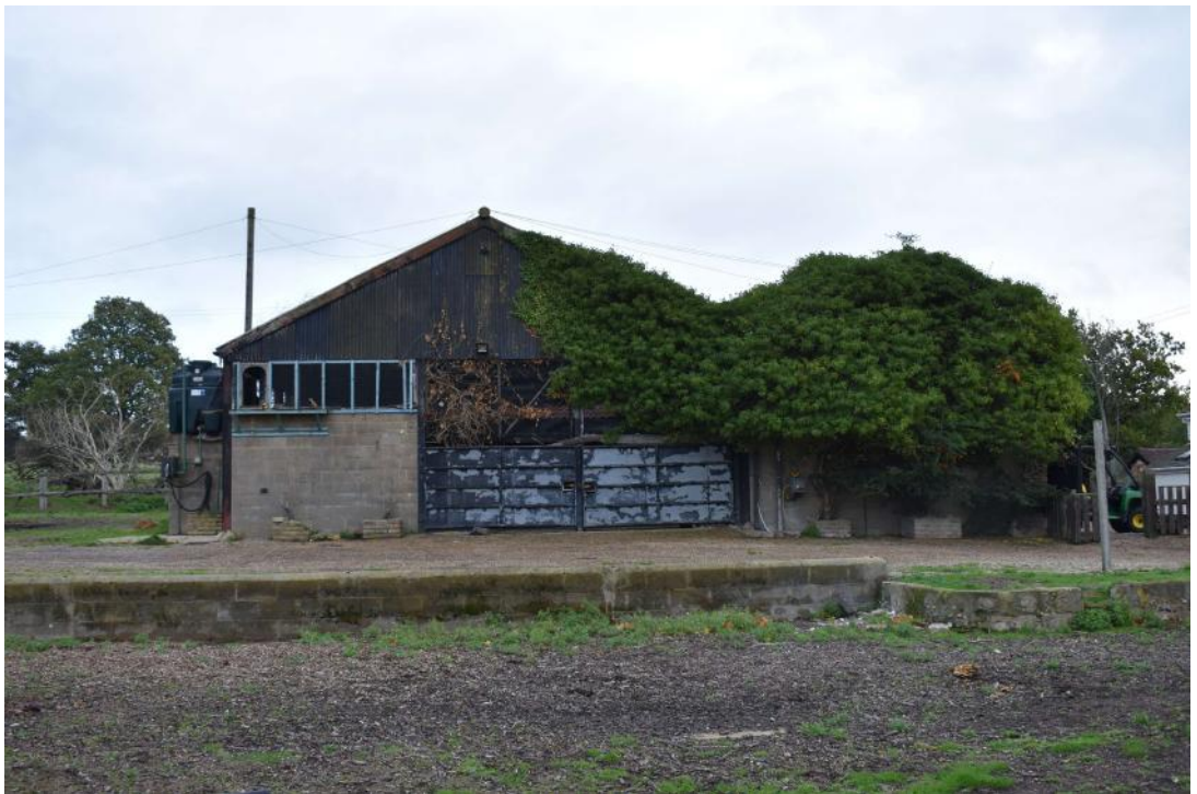
Photograph 3 South-west elevation. Photograph taken facing north-east.
