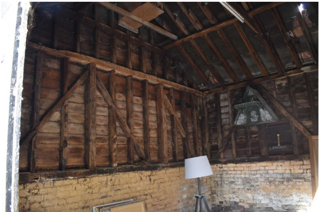
Photograph 10 Interior of Store 2. Photograph taken facing north-west.
