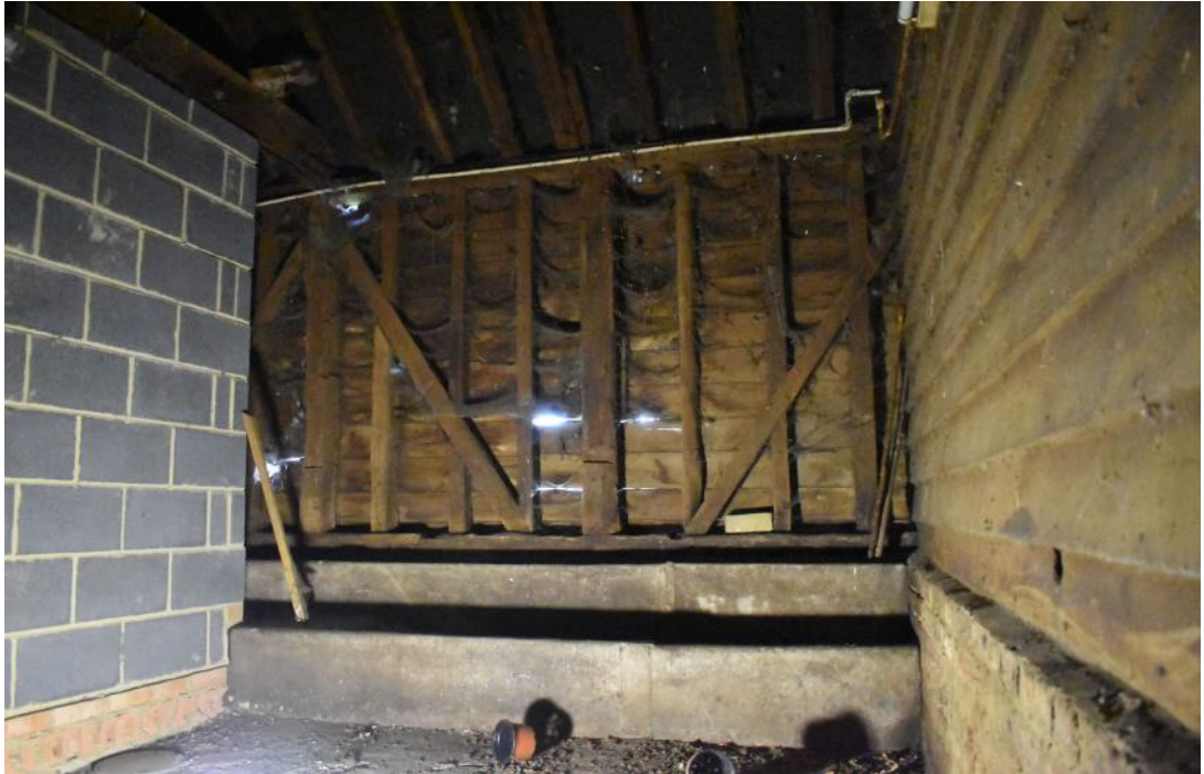
Photograph 13 Interior of Store 4. Photograph taken facing north-east.
