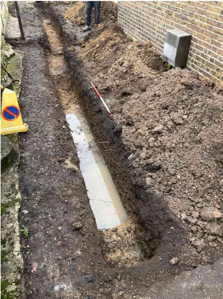
Photograph 2 Pit/pond F1, looking west-north-east.
