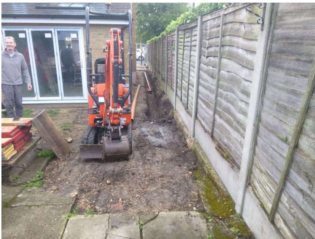
Photograph 4 Service trenches, looking east-south-east.
