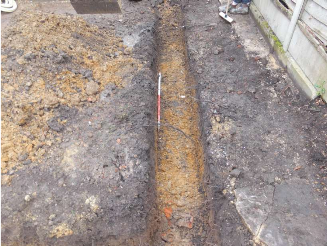
Photograph 1 Foundation trench, looking east-south-east.
