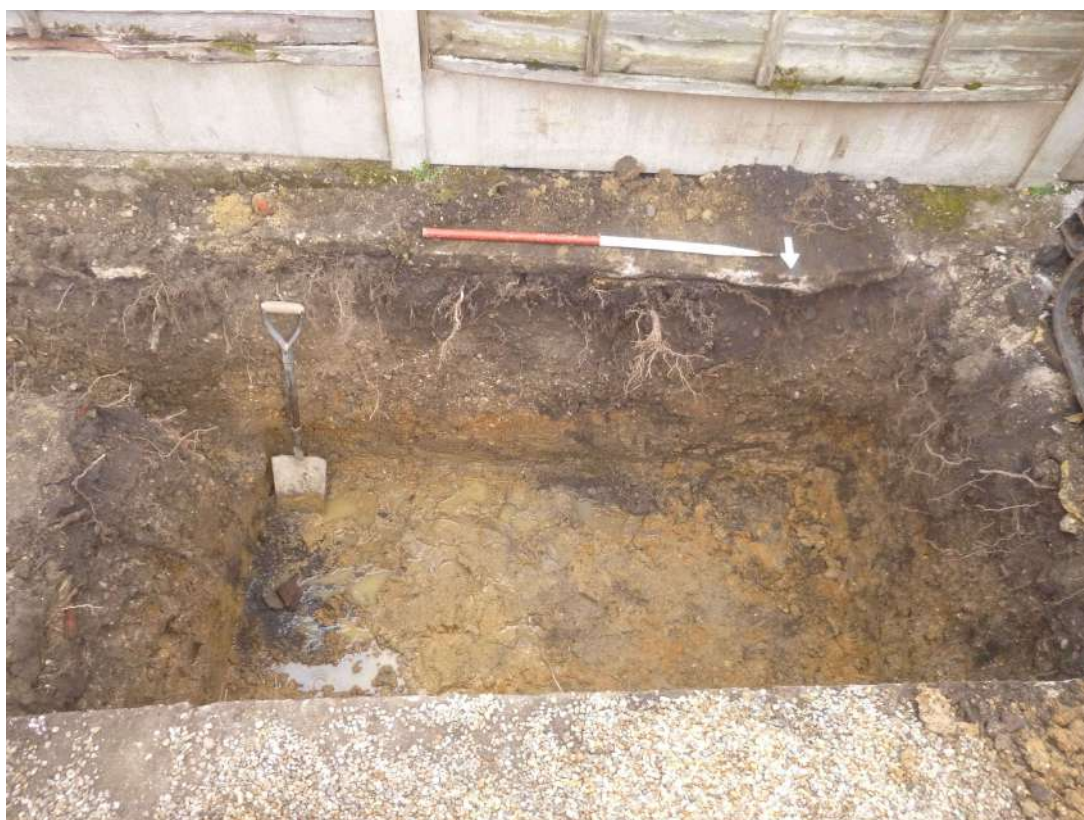
Photograph 5 New soakaway, looking south.
