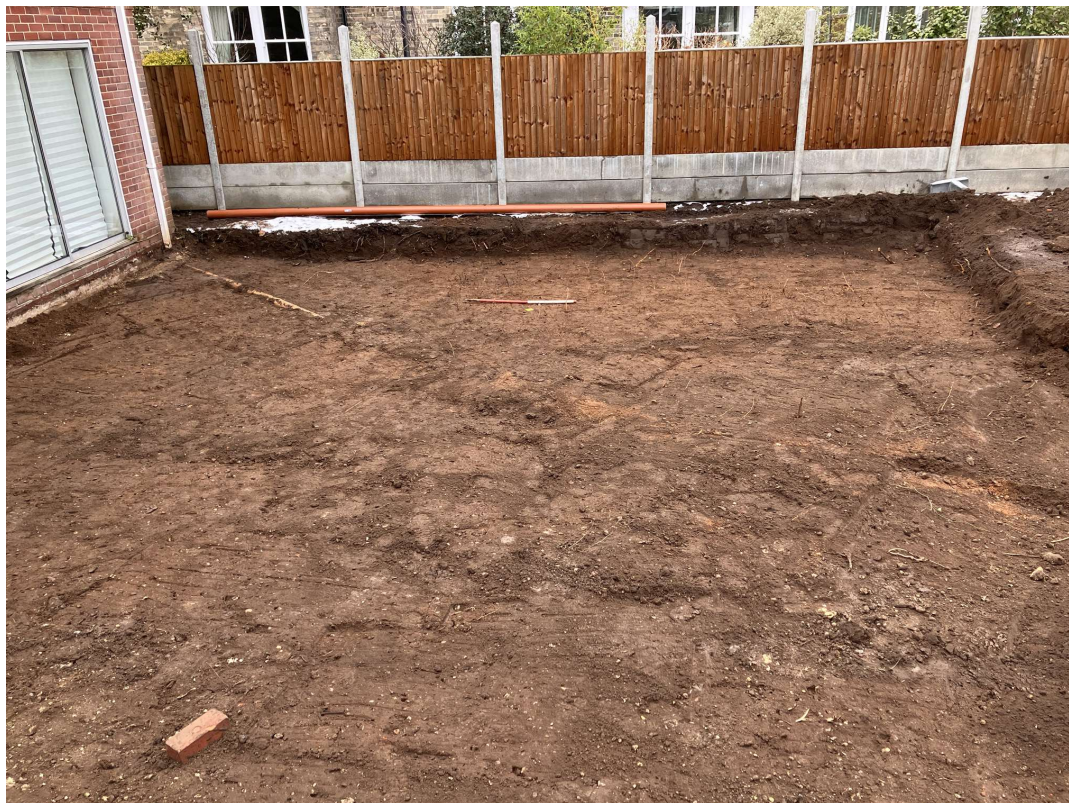
Photograph 2 Ground reduction area, looking west.
