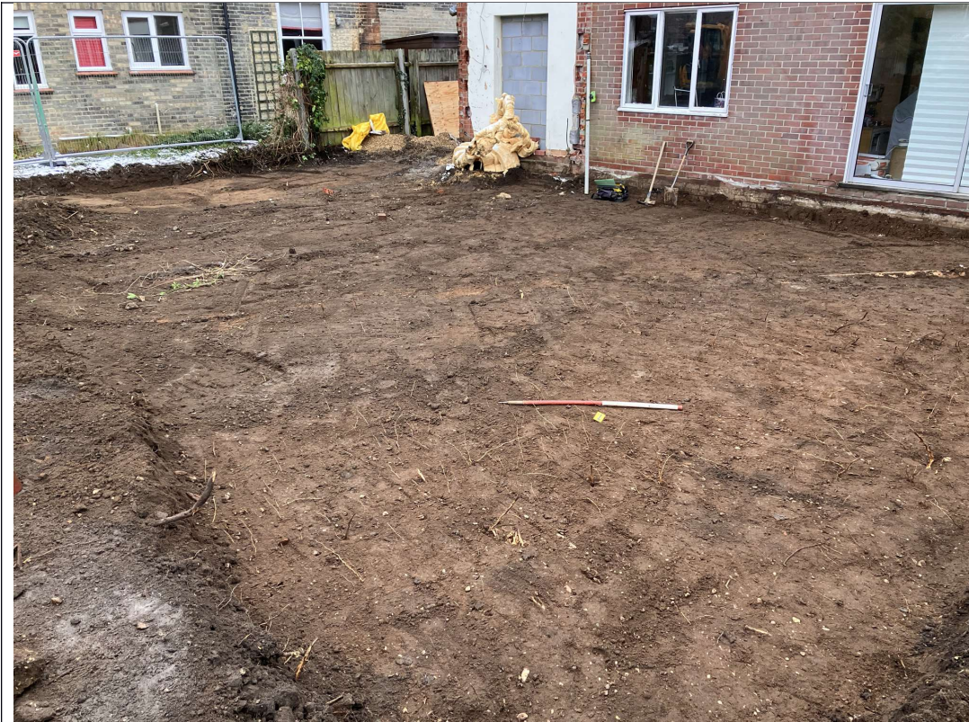
Photograph 1 Ground reduction area, looking south-east.
