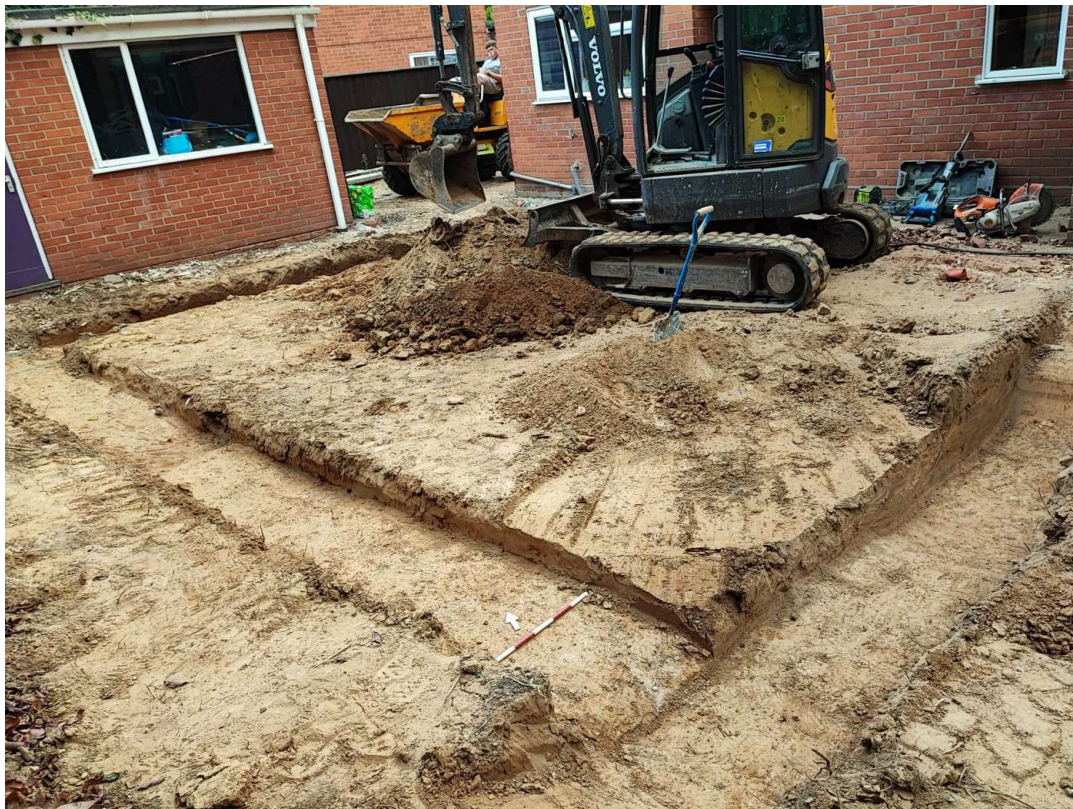
Photograph 3 Site shot showing foundation trenches, looking north-east.
