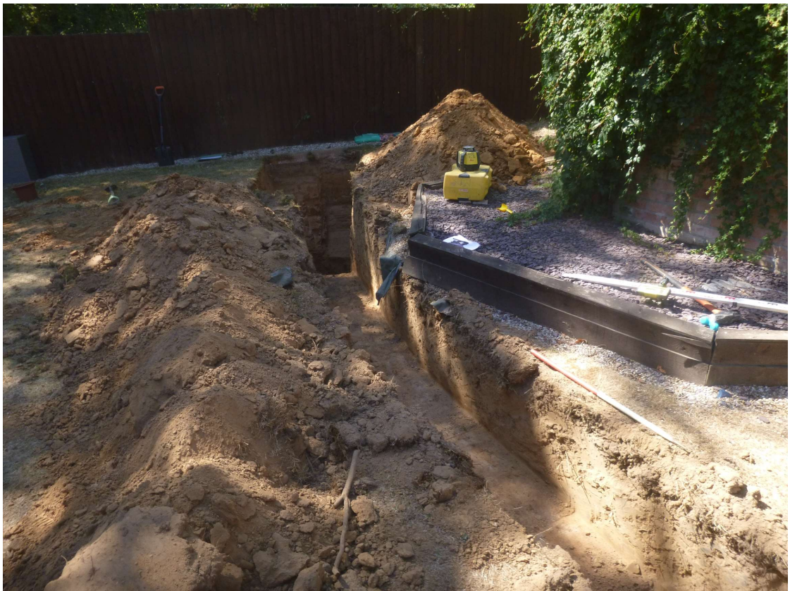
Photograph 2 Site shot showing drainage trench and soakaway, looking south-west.
