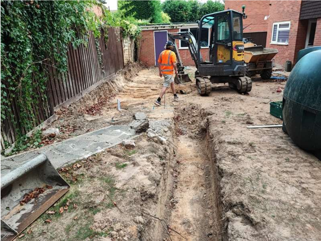
Photograph 1 Site shot, looking north.
