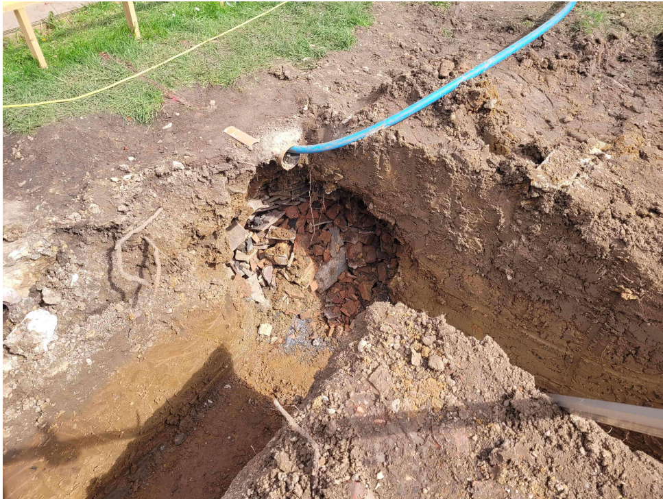
Photograph 2 Soakaway in north-eastern corner of foundation trenches.
